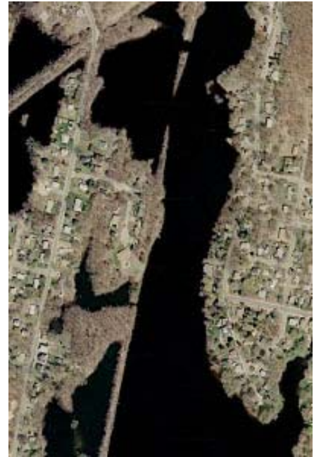
Figure III.3: ROW embankment across Harris Pond
