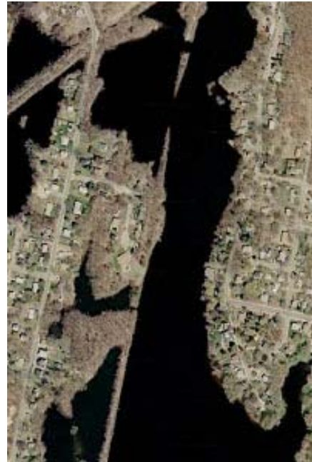
Figure I.5: ROW embankment across Harris Pond
