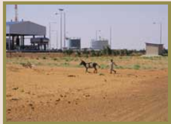
► Pump station 3 at El Munawara.
