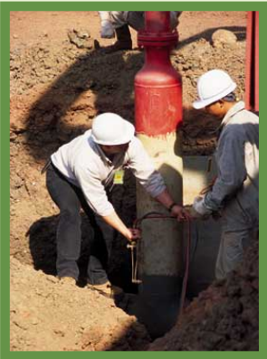
▶ Heglig HSE supervisor demonstrates proper safety technique.
