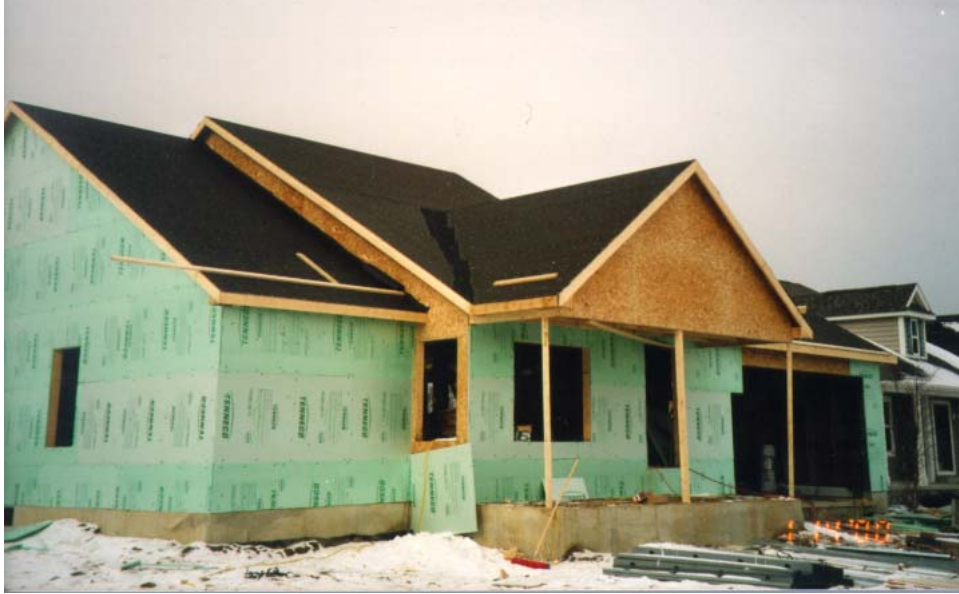
Steel House Sheathed with Rigid Foam Insulation
