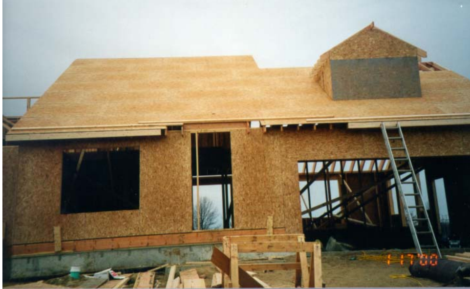
Framed Wood House
