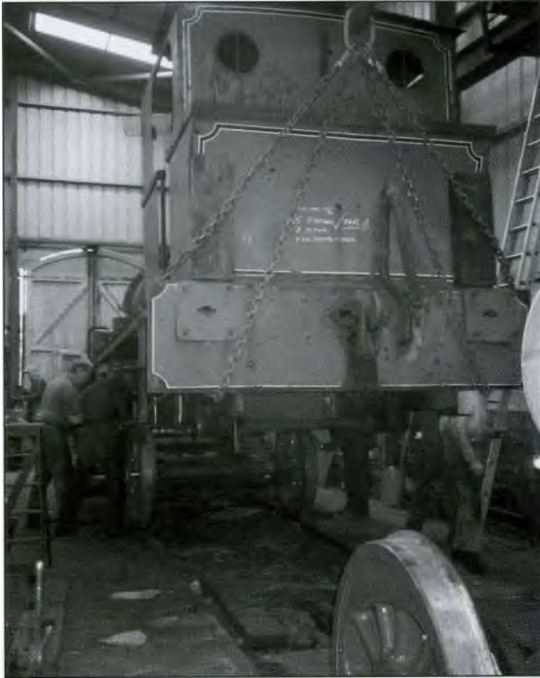
With its front end supported on blocks, No.3 is now raised to enable the wheelsets to be rolled into position. [J Wolseley]
