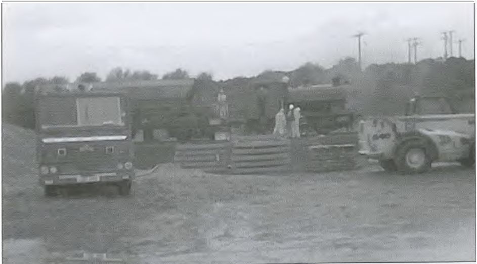
Water, water everywhere..... Fire Service assistance at Salt Mines. [A Ragg]
