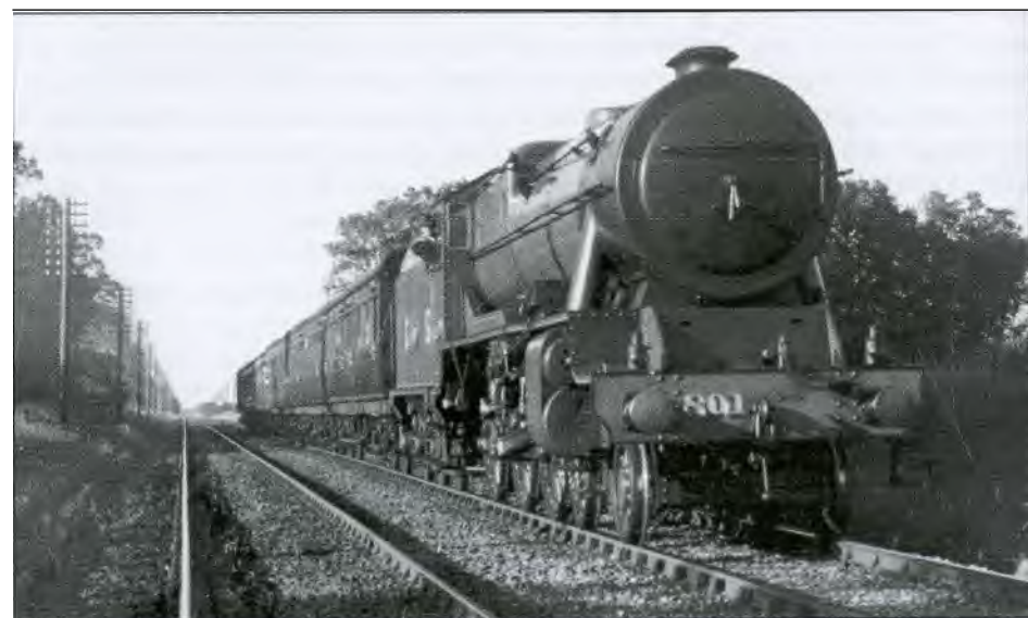
No.801, as yet un-named, with a test train near Templemore in 1940. A bowler-hatted inspector is in the fireman's seat and below him the drive for a speedometer can be seen mounted under the running plate. Can anyone comment on the coach behind the engine? [S Kennedy]
