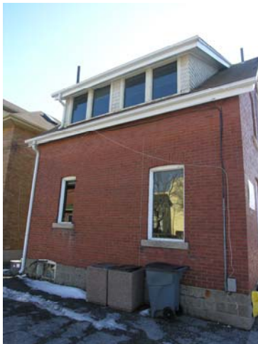
Figure 5 – 131 Trafalgar Rd., view of east (rear) façade
