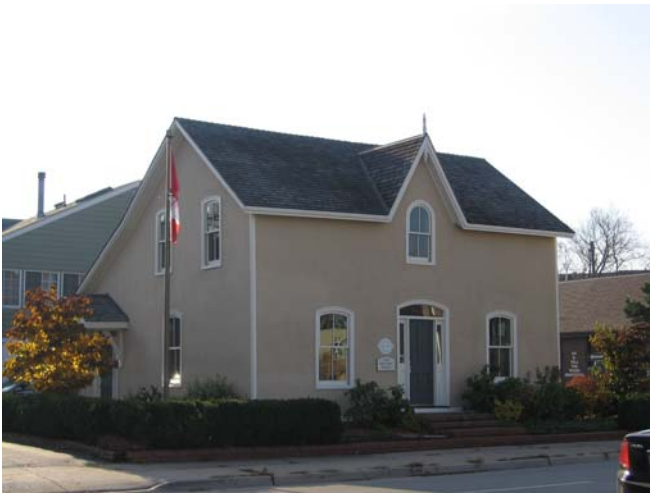
Figure 25 – 140 Trafalgar Rd., view of east (front) façade of the historically-designated building on the southwest corner of Randall St., premises of David Forman, Innkeeper, 1833
