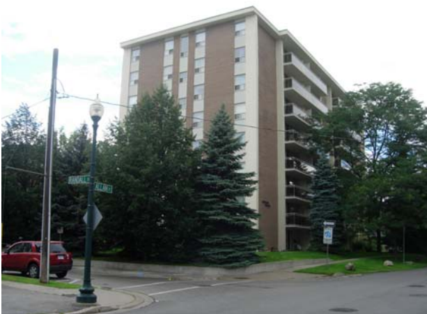
Figure 30 – Apartment building, 8 storey 150 Allan Street
