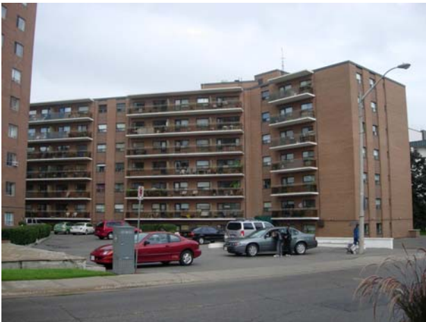
Figure 28 – Shoreacre Arms, 7 storey 105 Allan Street
