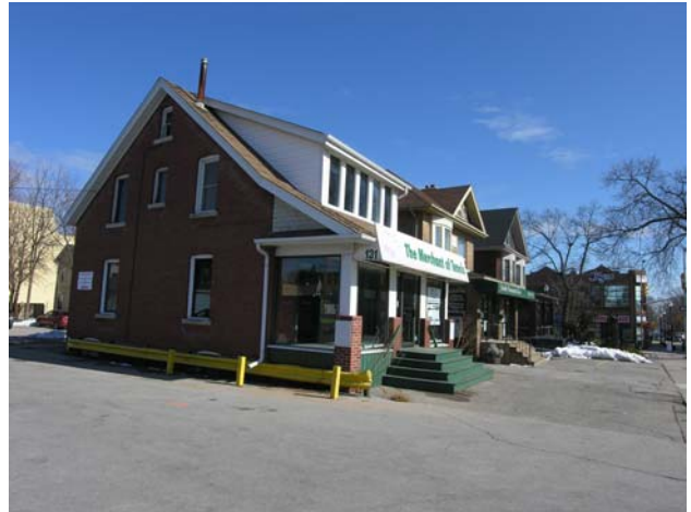
Figure 15 – 131 Trafalgar Rd., view of west (front) façade in context with its adjacent Edwardian house structures
