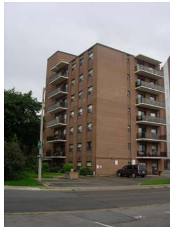
Figure 29 – Commodore Apartments, 7 storey 135 Allan Street
