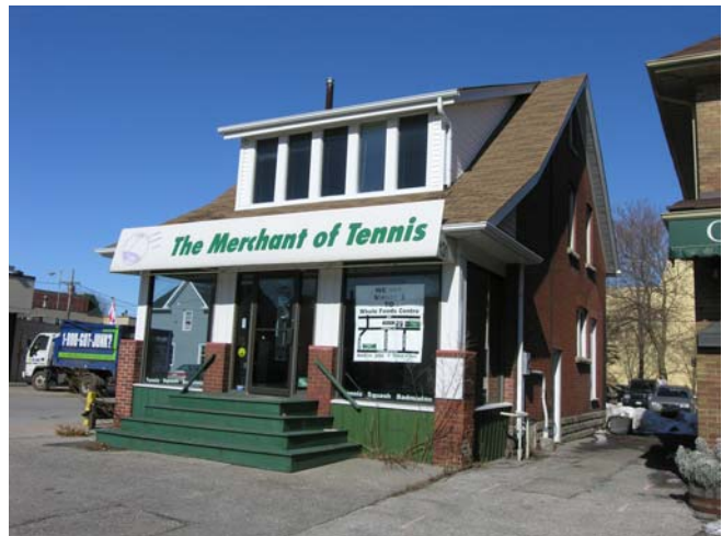
Figure 6 – 131 Trafalgar Rd., view of south (side) & west (front) façades
