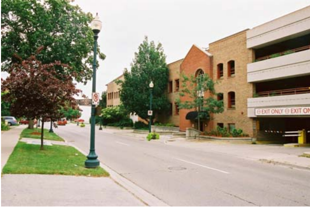
Figure 27 – 284-308 Church St., north (entrance) façade of municipal parking garage, 2 storeys
