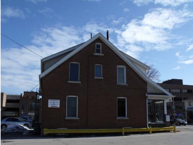
Figure 14 – 131 Trafalgar Rd., view of north (side) façade
