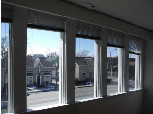
Figure 19 – 131 Trafalgar Rd., detail view of interior of front (west) dormer windows showing casing
