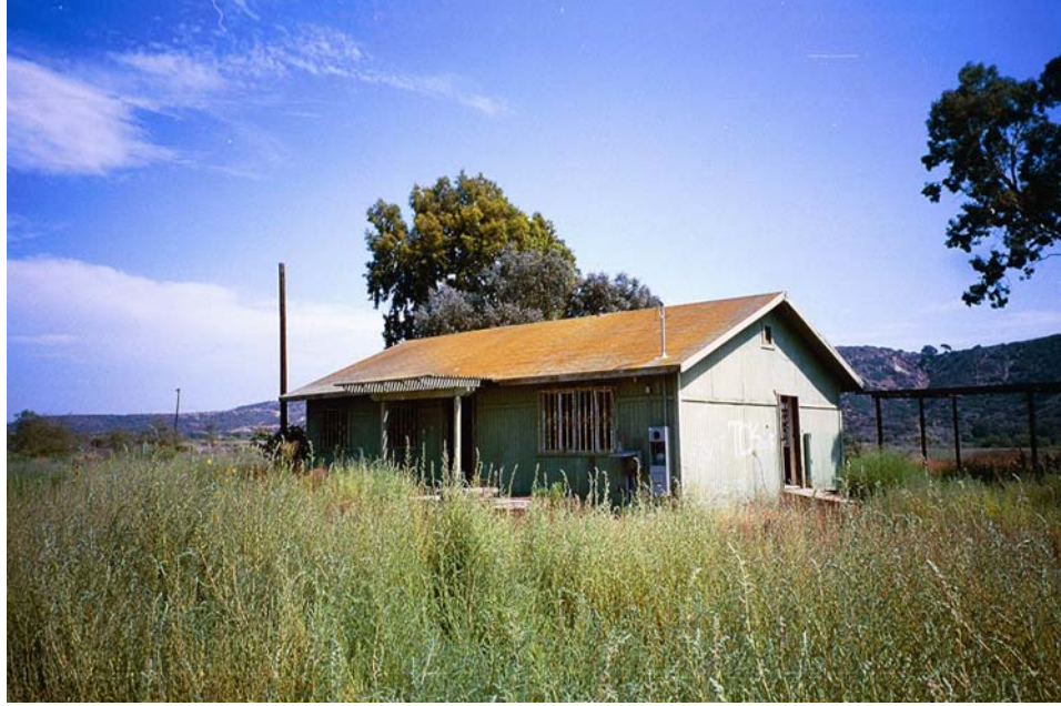
Photo 1.4.5.2-1. Resource TJ-4H, facing southeast.
