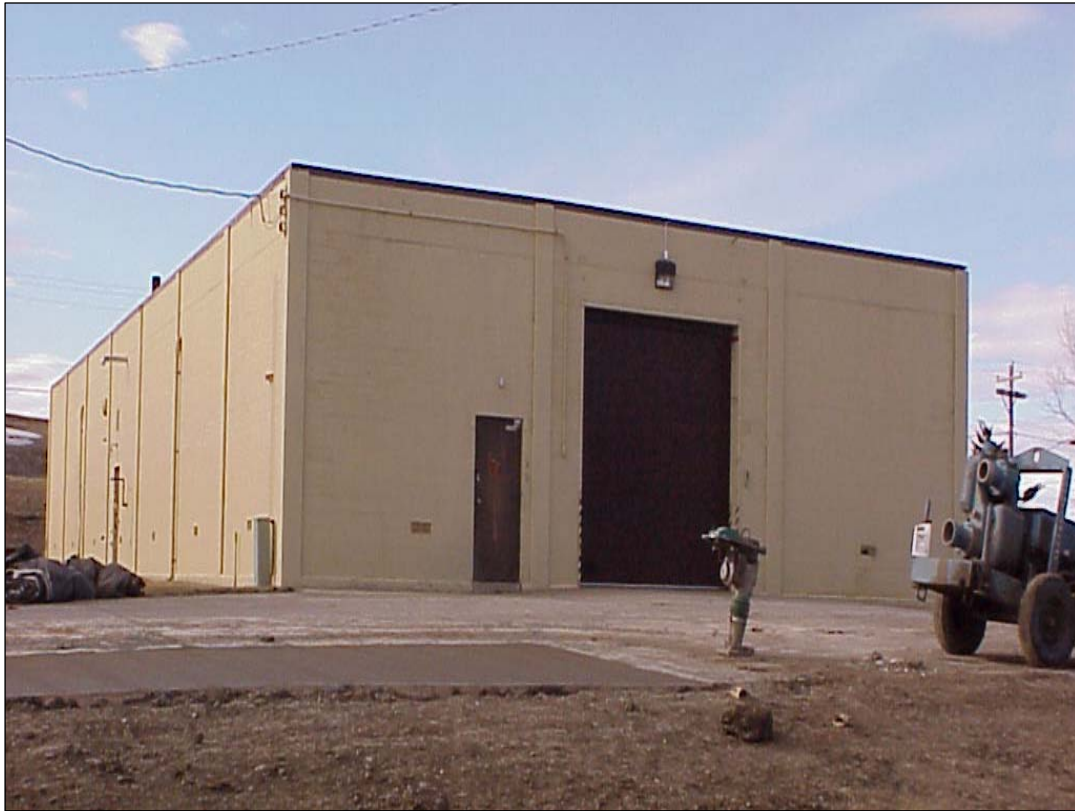
Building 88323 - storage facility for inert spares
