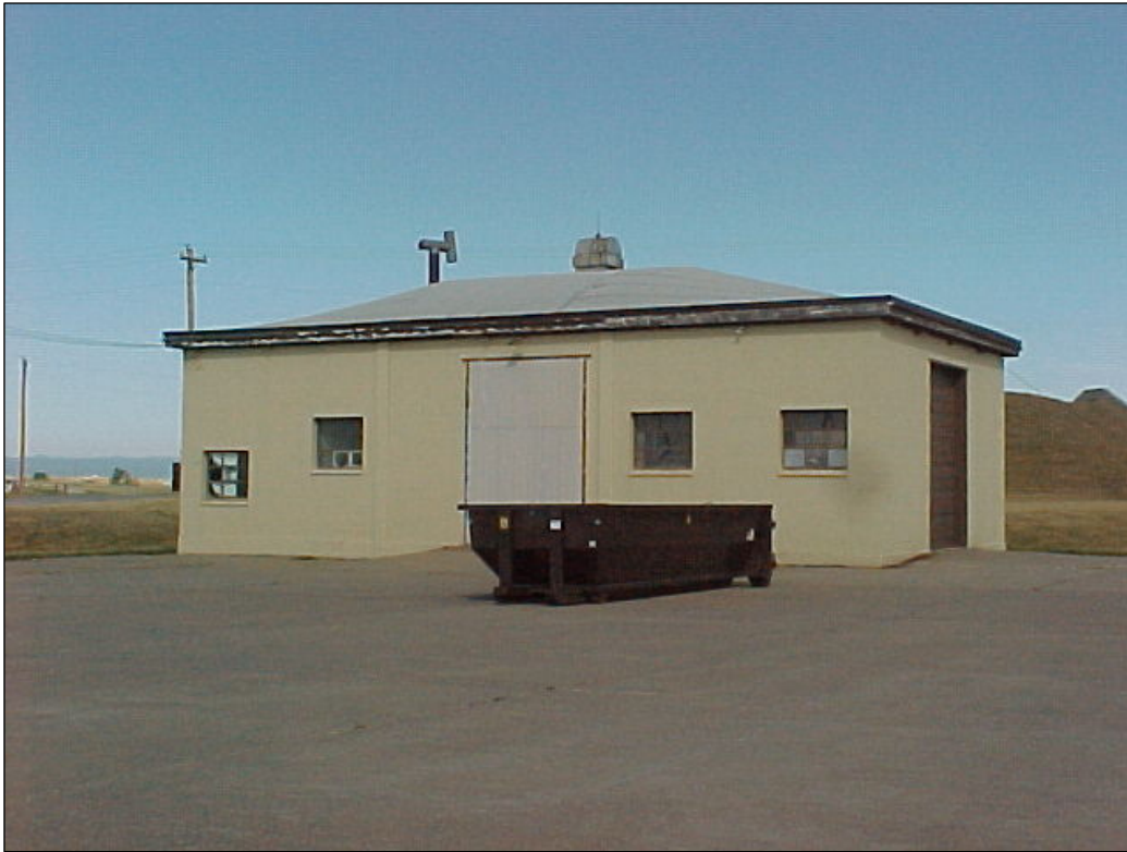
Building 88030 - Warehouse, Supplies and Equipment Building
