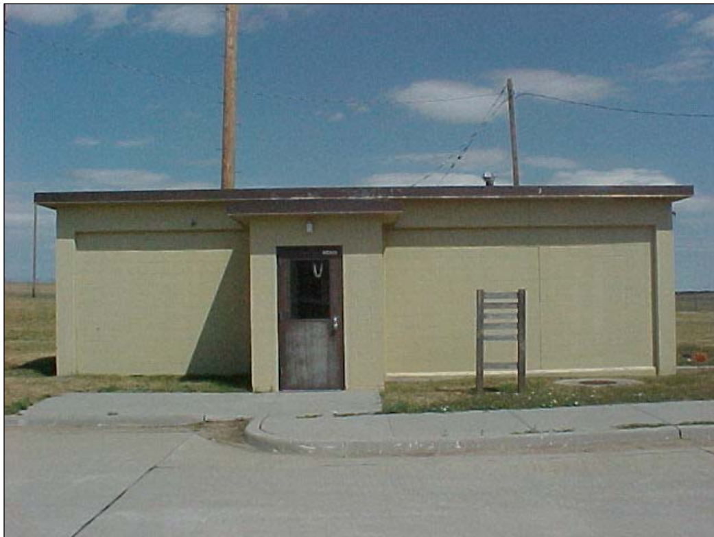
88320 - Crew Readiness Building
