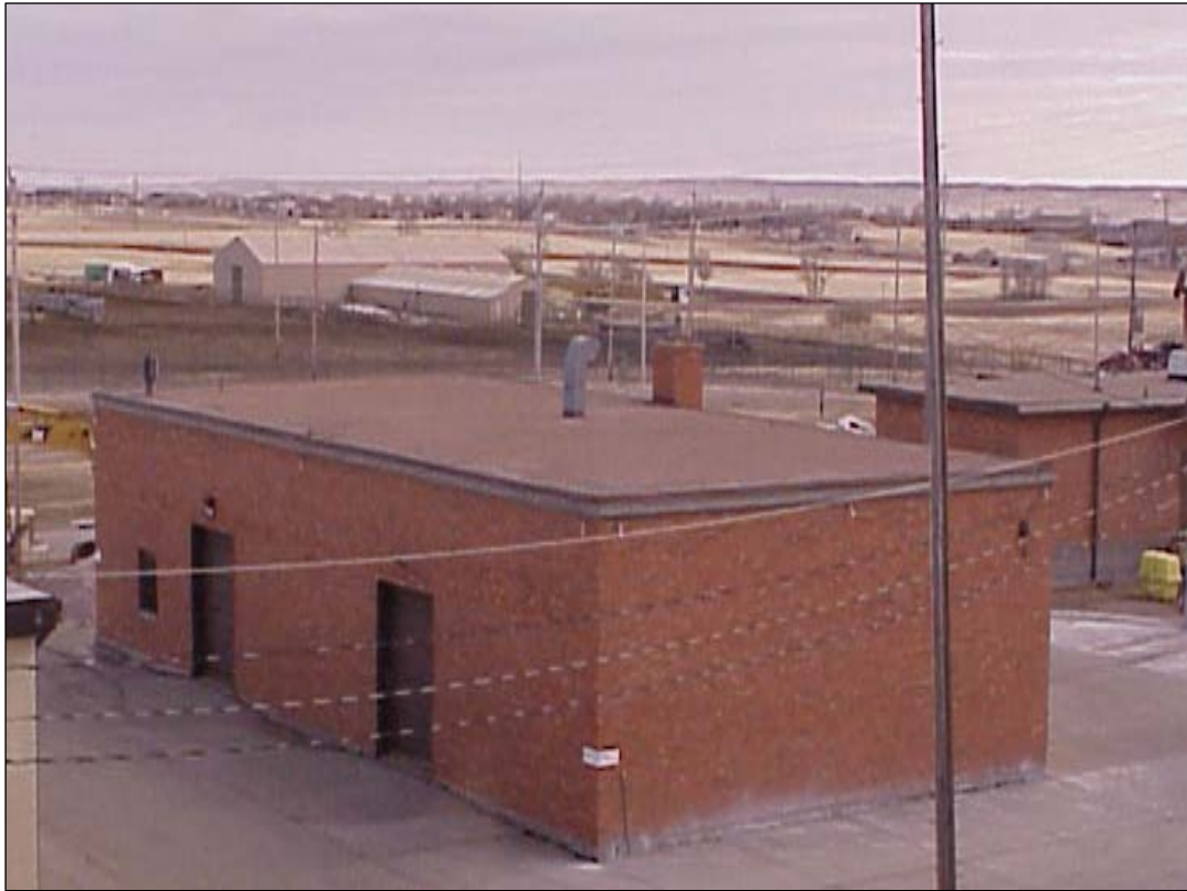
Building 88315 - storage facility for inert spares
