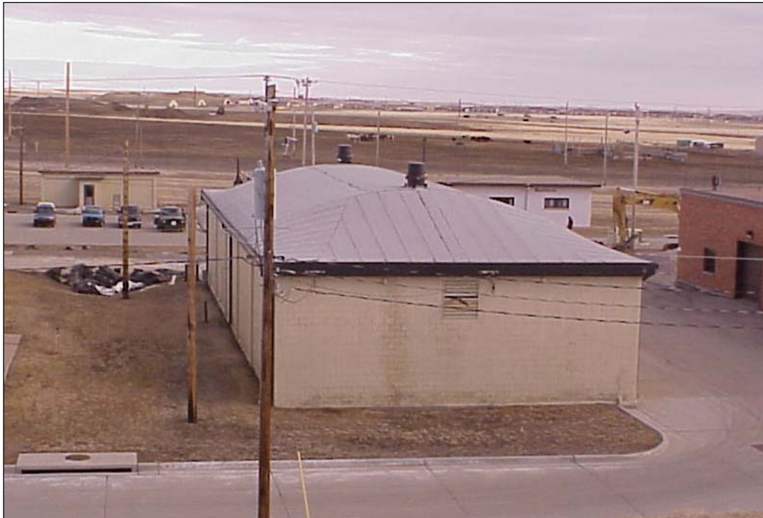
Building 88319 - storage facility for inert spares
