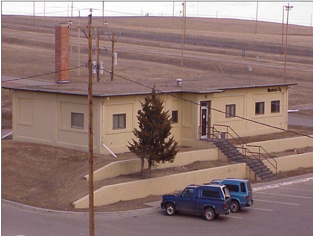
Building 88327 - communications operation facility
