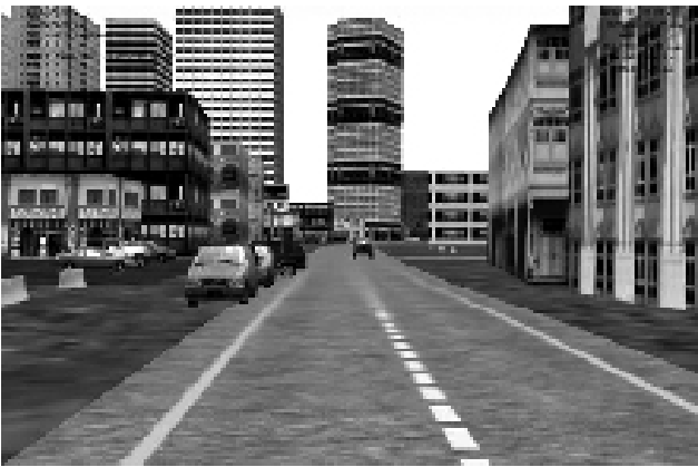
Figure 7. Street level view of AOI
