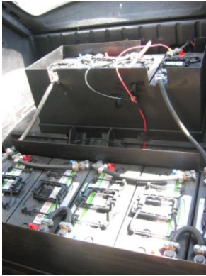
Figure 13. Battery boxes fabricated, batteries installed and connected in series.
