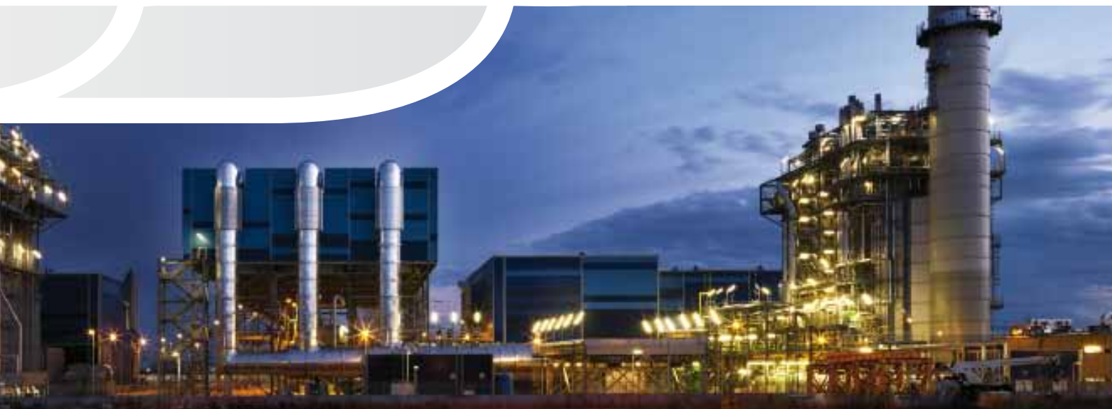
Finmeccanica - Combined Cycle Power Plant, Rizziconi, Reggio Calabria
