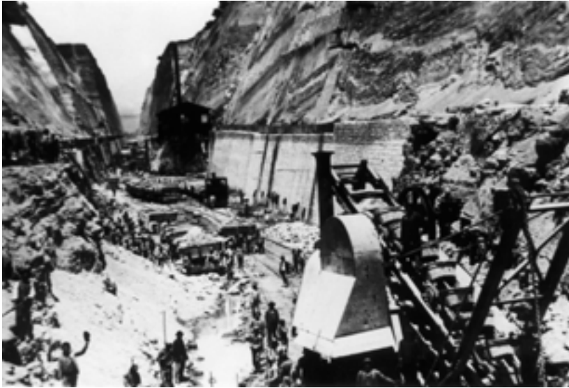
Fig. 126: Work in progress at the Corinth Canal ca 1885, a decade before Boland crossed it.
