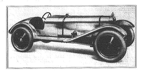
The 1926 Alvis 12/80 supercharged front wheel drive car offered at £1,000 and guaranteed to lap Brooklands at 100 mph. What a stunner.
