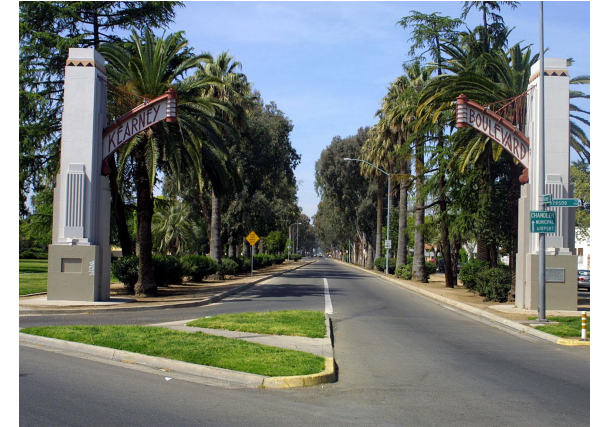
The realignment of Kearney Boulevard at Fresno Street would add public space to facilitate the civic uses described on page 20.
