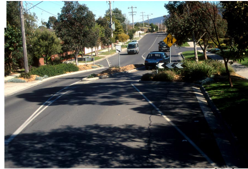
Angled slow points include extended curbs on the edges and a median between lanes. Drivers slow down to maneuver the curve this creates.
