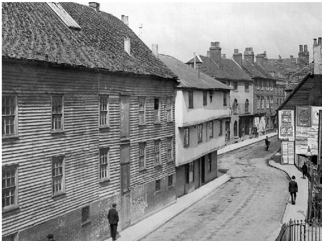
Mill Street prior to widening to accommodate tram lines.
