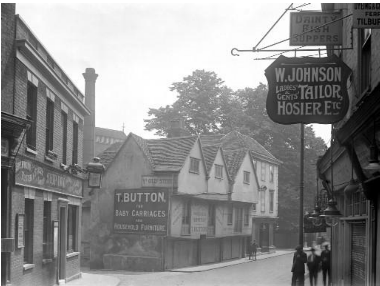
The chimney of the Lower Brewery can be seen in the background of this old photograph of the bottom of Gabriel's Hill.
