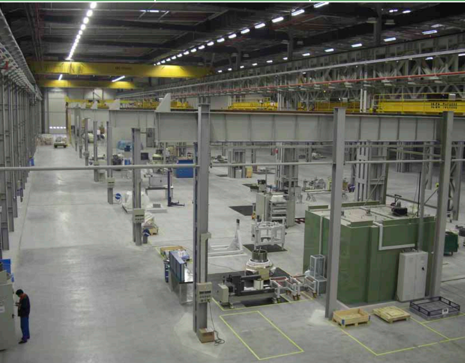
Interior view of Hansen's wind turbine gearbox plant in Tianjin – China. First gearbox delivered in March 2009.
