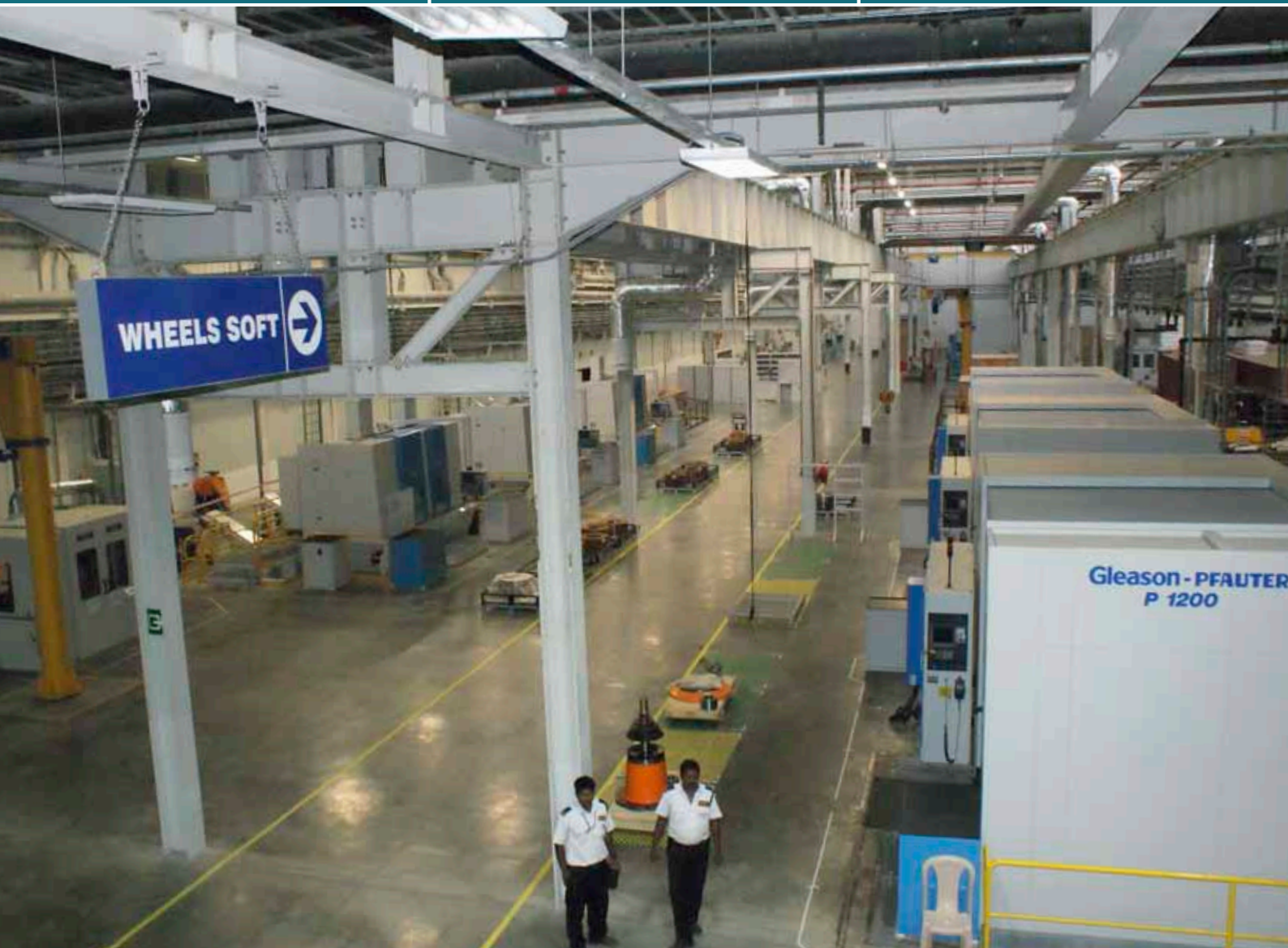
Interior view of Hansen's dedicated wind turbine gearbox plant in Coimbatore – India. First gearbox delivered in September 2008.
