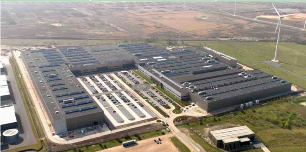
Hansen's dedicated wind turbine gearbox plant in Lommel – Belgium.
