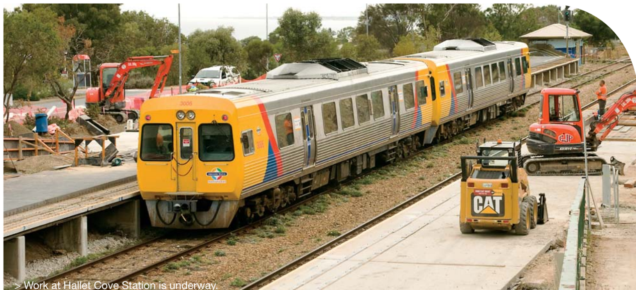
> Work at Hallett Cove Station is underway.
