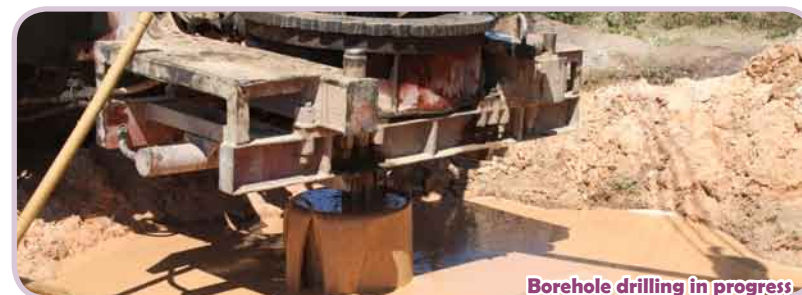
Borehole drilling in progress
