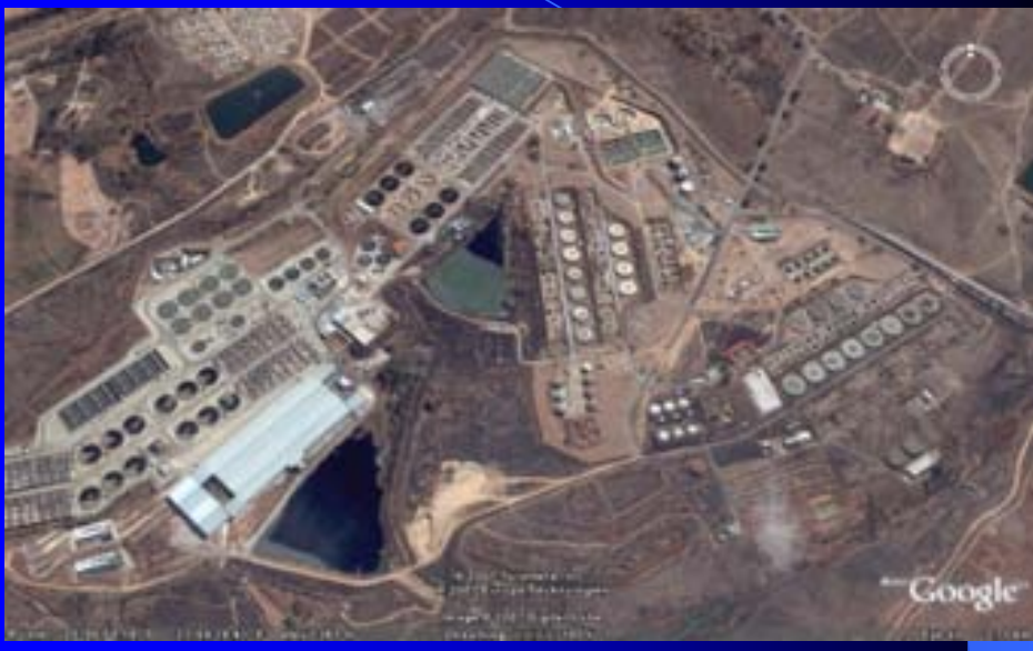
Northern Sewage Works - waste water treatment plant
