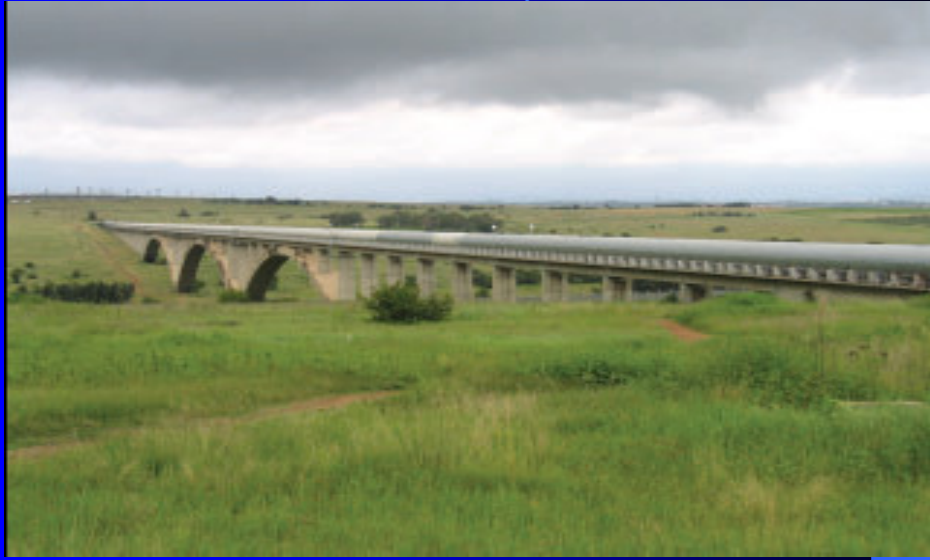
Sewage pipeline from urban metropolitan to Northern Sewage Works
