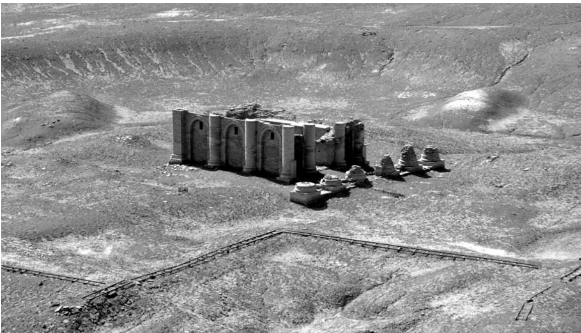
Fig. 25. Aerial view of the restored Gareus Temple
