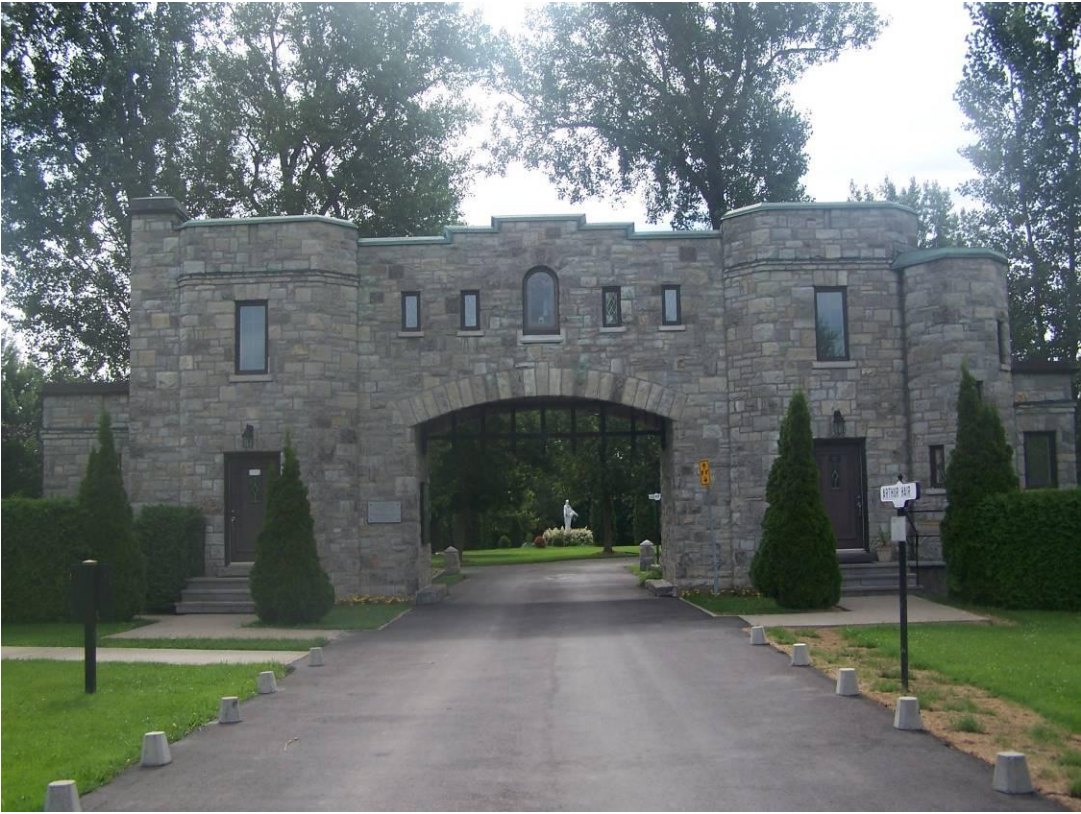
(Fig 7-View of South and North tower as it shall be referred to throughout the paper for easier understanding)
