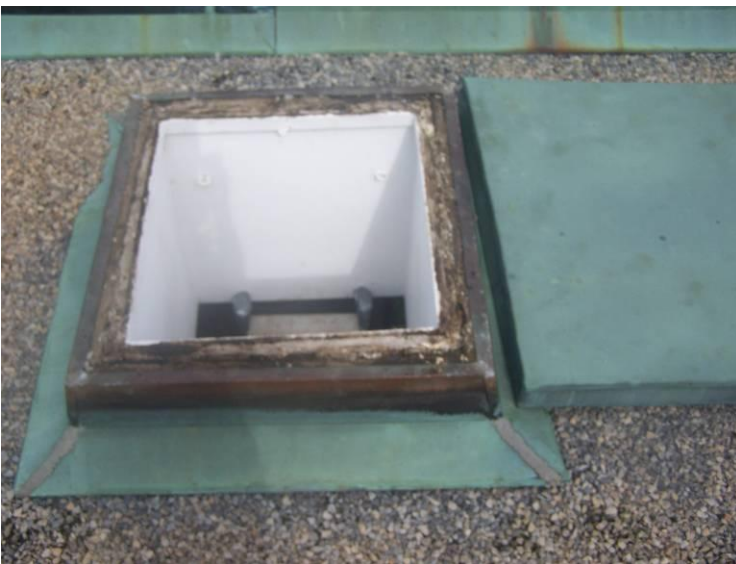
(Fig 19-Ceiling hatch to access the roof)
