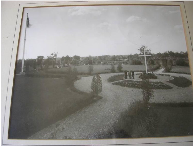
(Fig 1-Space on the road before the construction of the Gate)
