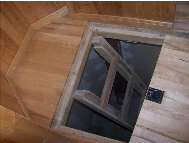
(Fig 15-Trap door leading to basement and the remnants of the staircase circle)
