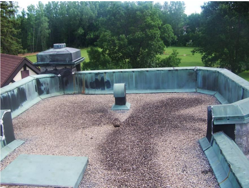
(Fig 4- Gravel and tar roof with copper siding)
