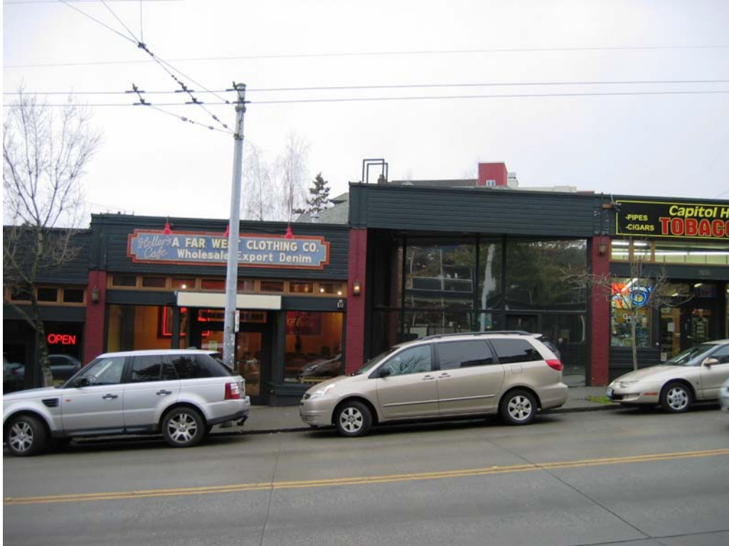
Figure 25 – E. Olive Way elevation, 2009
