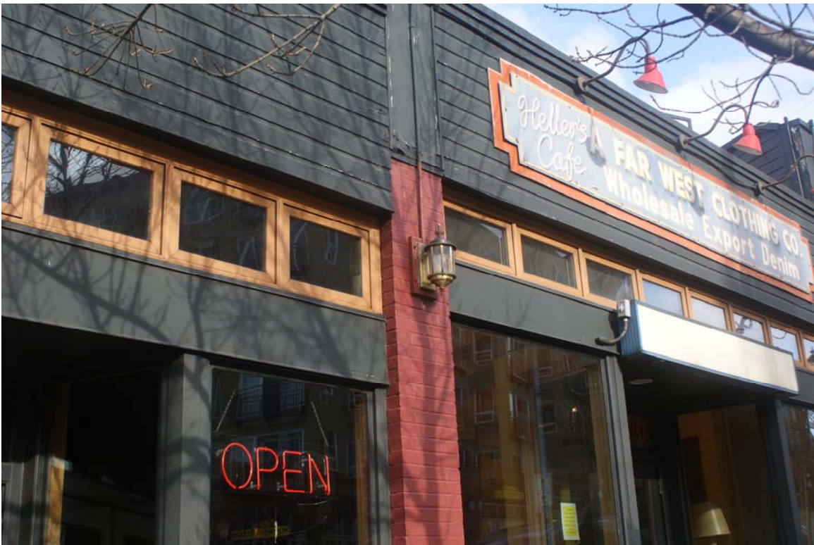
Figure 28 – E. Olive Way elevation, detail, 2009
