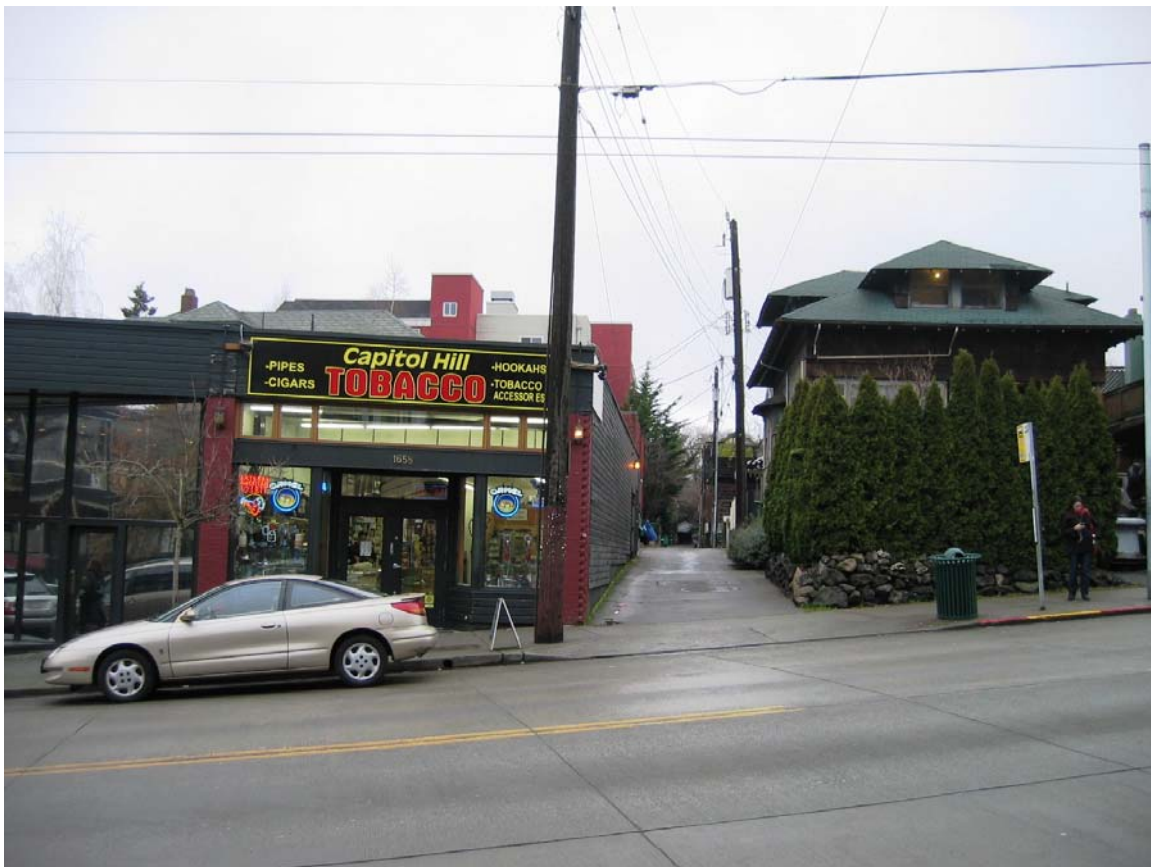
Figure 26 – E. Olive Way elevation, 2009
