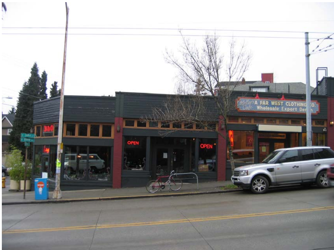
Figure 24 – E. Olive Way elevation, 2009
