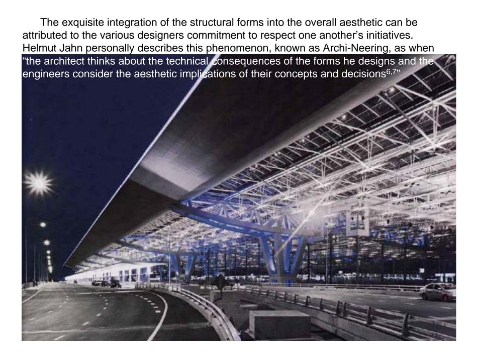
When these methods are applied to Suvarnabhumi, the result is structure in its most efficient form. In fact, the function of each individual truss is expressed explicitly in its form, and thus "structurally rationalist" in nature. The eight composite 2,710-ton trusses supporting the canopy of the Main Terminal are "essentially diagrams of the bending moments acting on them, with the greatest depth at midspan and over the supports<sup>6</sup>." The differing cross sections can be seen below.
