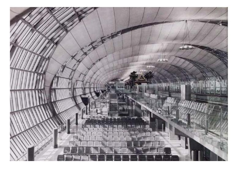
One should not be fooled by the apparent simplicity of Suvarnabhumi's floor plan (shown right). Rather, the Suvarnabhumi Airport is a dynamic structure with trusses of varying cross sections and composite constructions that effectively fuse design and structure.
