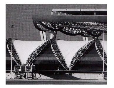
Though a different structural system from that used in the Main Terminal, the fivepoint truss achieves the same end: an open floor plan devoid of columns.
