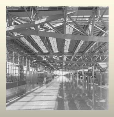
The use of two chords to combat compression provides additional benefits beyond mere reinforcement. By spreading the chords out to either side of the neutral axis, the Moment of Inertia is increased (increasing the stiffness of the cross section). In addition, the resultant triangulation of the cross section creates an opportunity for the trusses to effectively interlock into one mega-truss (this connection is shown above).
