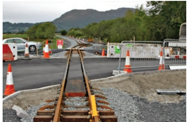
▲ On 7th September, at Pont Croesor the track is fully over the bridge, across the road and over the new entrance to the Osprey Centre. On the next stretch, track is down on the ballast, with the turnout for the proposed loop in place and all awaiting final alignment. All: John Stretton
