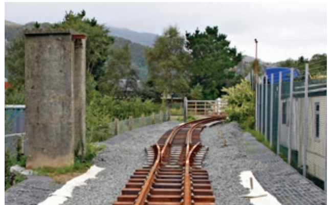
▲ On 7th September, at Pont Croesor the track is fully over the bridge, across the road and over the new entrance to the Osprey Centre. On the next stretch, track is down on the ballast, with the turnout for the proposed loop in place and all awaiting final alignment. All: John Stretton
