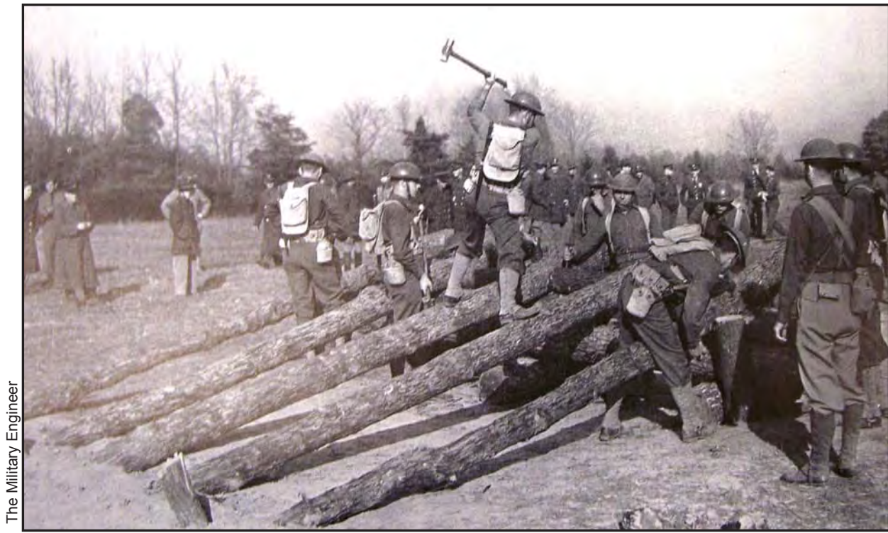
Men of the 5th Engineer Regiment build an antitank log crib at Fort Belvoir, VA.
