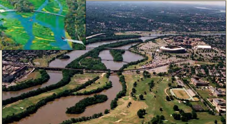
Simulated photo of Kingman Island and the Anacostia River showing the construction of wetlands (bright green areas) along its banks.
