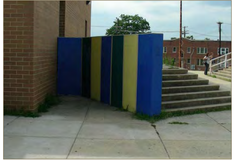
The broken sight lines on the grounds of some elementary schools, like the one here blocked by an outdoor stage, present safety issues even during daylight hours.
