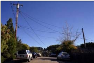
Visible overhead utility lines
