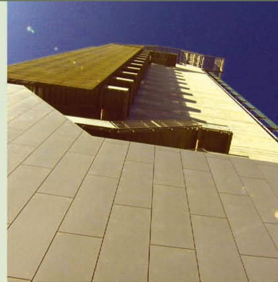
Exterior building façade © Rocky Mountain Institute
