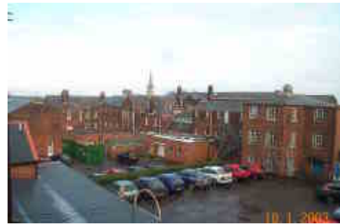
Administration/dining/chapel and kitchen range. Buildings form the core of the workhouse and constitute a strong group. Southern most range, of limited architectural merit includes a flat roofed element.
