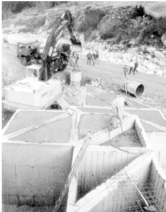
Figure 4.8. Massive precast concrete prisms placed as a groin field, Switzerland. (44)
