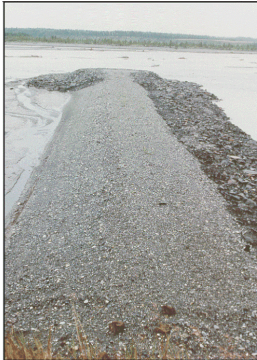
Figure 9.13. Impermeable spur field in top photograph with close-up shot of one spur in the lower photograph, vicinity of the Richardson Highway, Delta River, Alaska.
