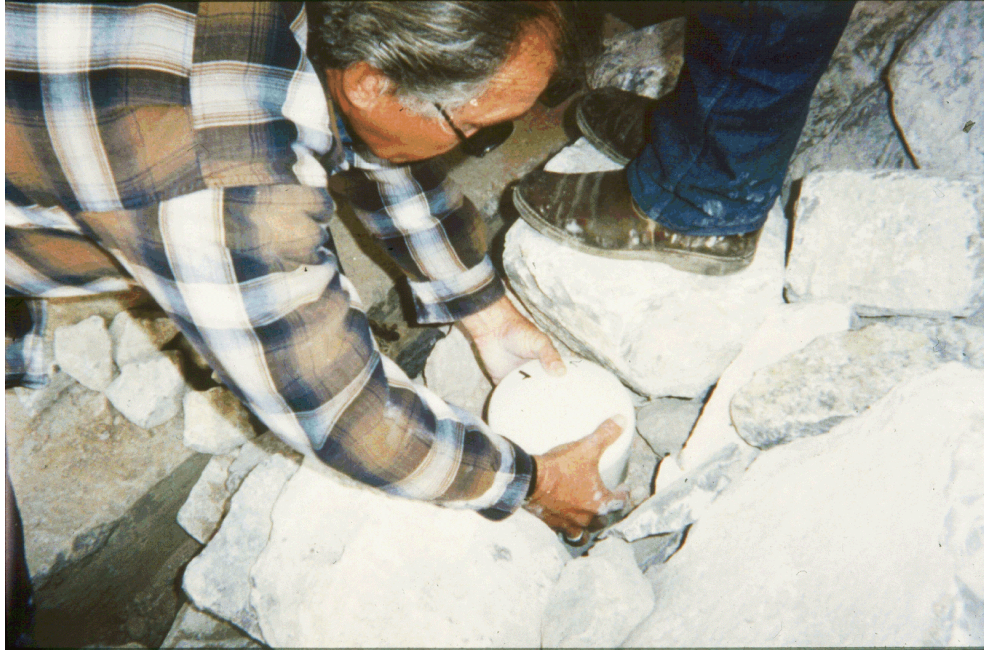
Figure 7.18. Installation of a float out device by Nevada DOT to monitor riprap stability.
