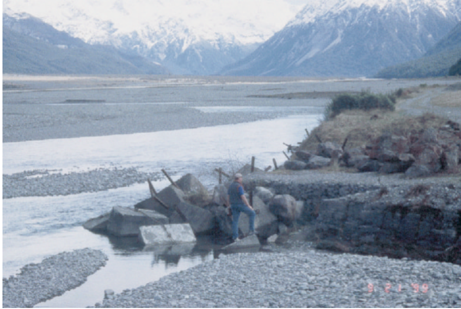
Figure 4.9. Concrete cube bank revetment, Waimakariri River, New Zealand. (45)
