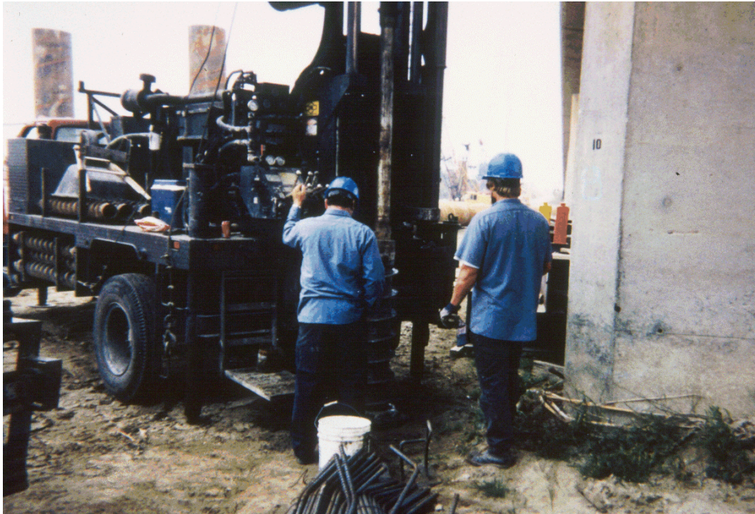
Figure 7.15. CALTRANS drilling with hollow stem auger for installation of float out devices at Salinas River bridge (Highway 101) near Soledad, CA.
