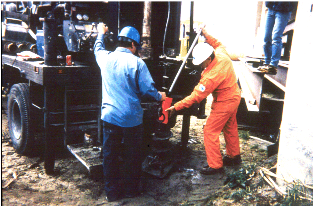
Figure 7.16. Installation of float out device on Salinas River bridge near Soledad, CA.
