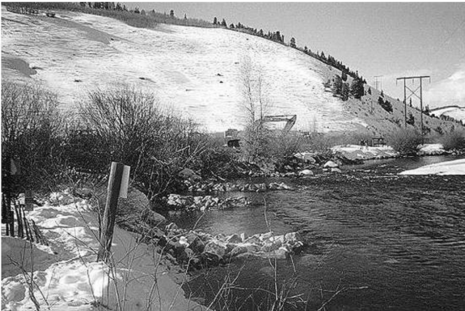
Figure 1.5. Bendway weirs installed on the Blue River near Silverthorne, Colorado (CDOT).
