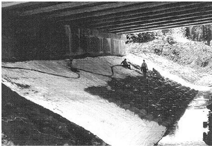
Figure 5.5. Installation of articulating grout filled mat proceeding upslope (ODOT). (6)
