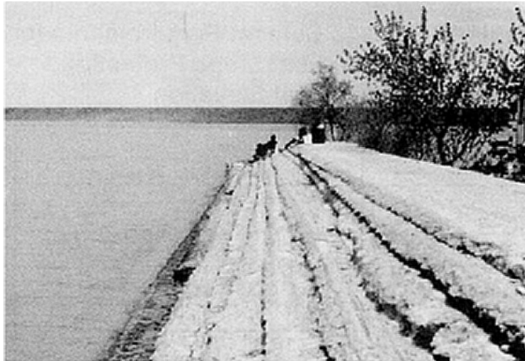
Figure 2.1. Stair step facing on Bonny Reservoir, Colorado after 30 years (PCA).
