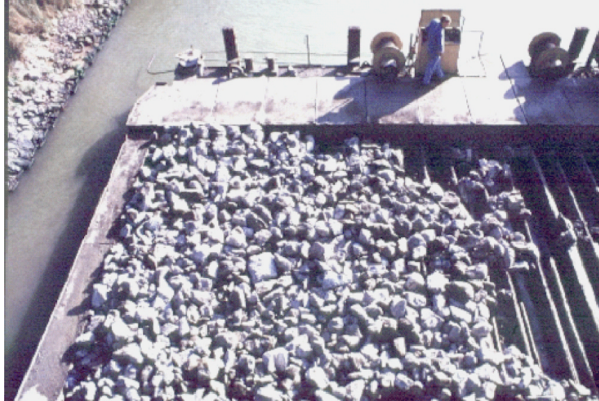
Figure 4.10. Bottom dump pontoon barge used in Germany for placing riprap. (32)
