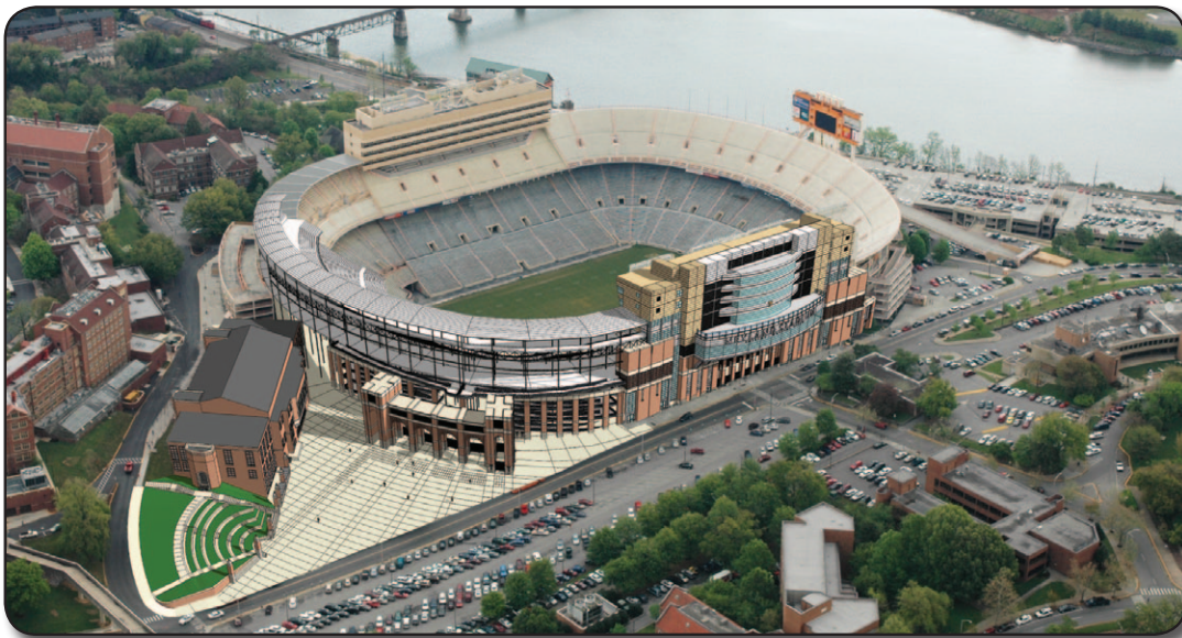
Phase III will include the west exterior facade and a new Gate 21 Plaza.
