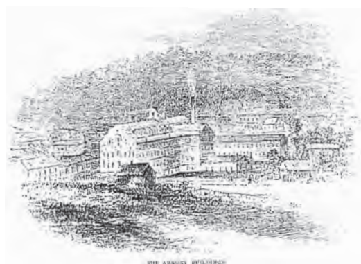
Figure 9. A sketch of the armory buildings on Franklin St. by T. Addison Richards, Harper's New Monthly , 1864.
