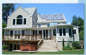
Home in Virginia with 80-gallon evacuated-tube solar water heater and 2.7-kW PV system. *Courtesy: Standard Solar*
