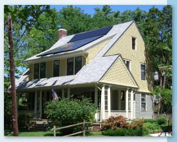
A 6-kW PV system provides 85 percent of this Washington, D.C. home's electricity. *Courtesy: Standard Solar*
