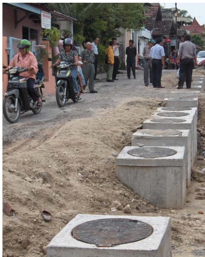
Drainage system construction in Blitar, East Java
