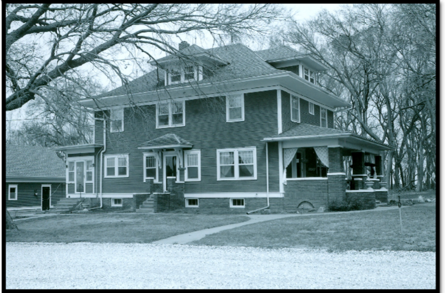
View: NW Photo by Stacy Stupka-Burda, 8 April 2008, NSHS
