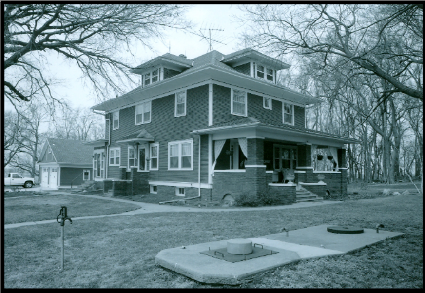
View: NW Photo by Stacy Stupka-Burda, 8 April 2008, NSHS
