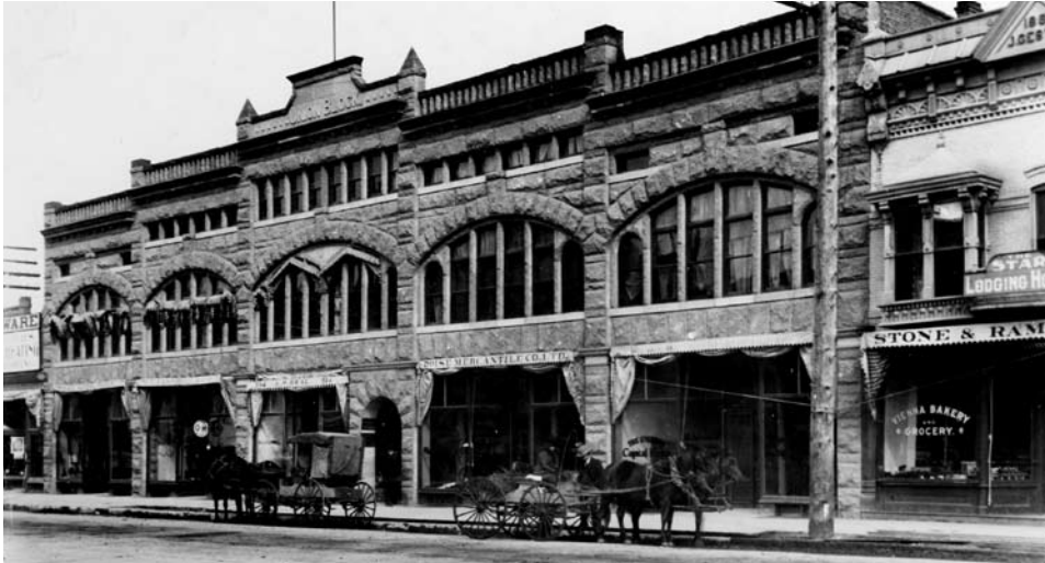
Above: The Union Block shortly after construction. ISHS No. 69-4.39
