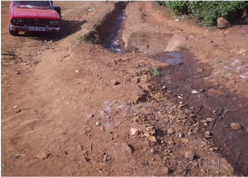
Fig 2: Storms drain being used to discharge waste water
