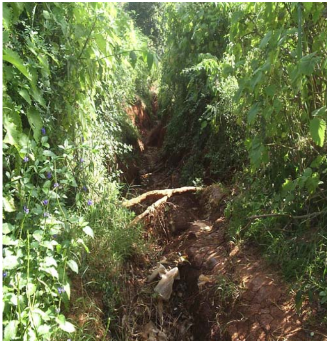
A road turned to a gully by runoff from the road and a banana crop on a cut off drain (COD) used to harvest road runoff.
