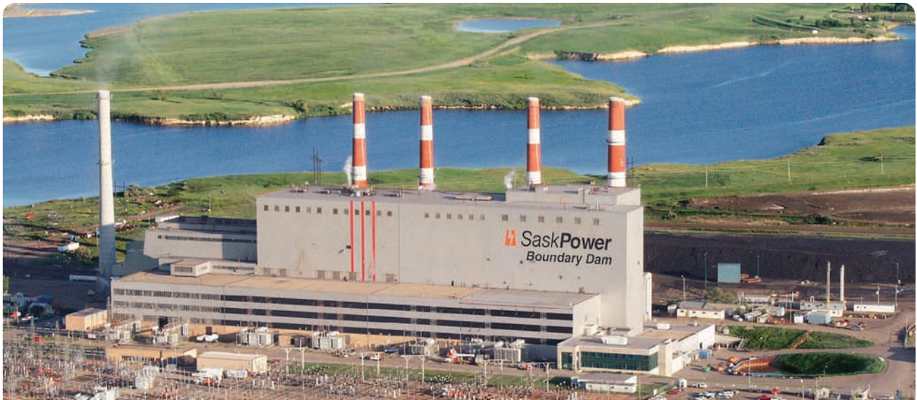
A decision on whether to proceed with the construction of an integrated carbon capture and storage system on Boundary Dam Power Station Unit #3 is expected to be made in 2011.
