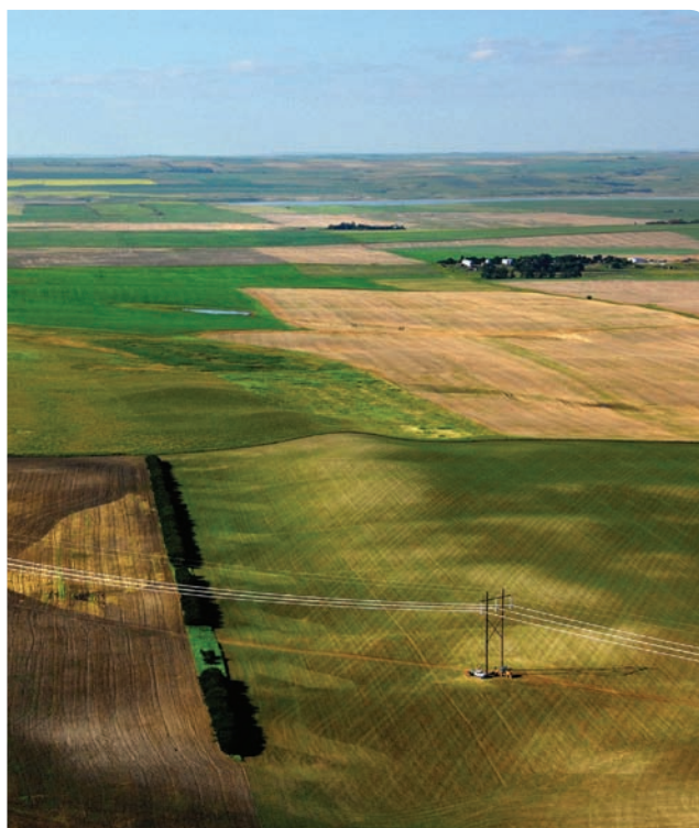
In 2010, SaskPower completed the design and construction of a 230-kilovolt transmission line from Poplar River Power Station to Pasqua Switching Station near Moose Jaw.
