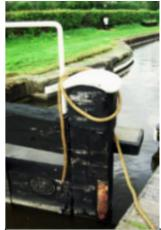
Figure 10 Handrail impeding safe use of strapping post on a lock gate
