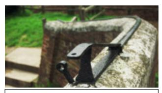
Figure 2 - The roller is lost but the guard iron remains in situ on this bridge parapet
