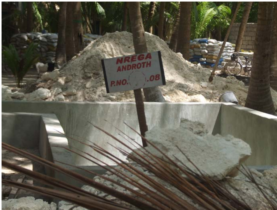
A pond construction under MGNREGA at Andrott Island
