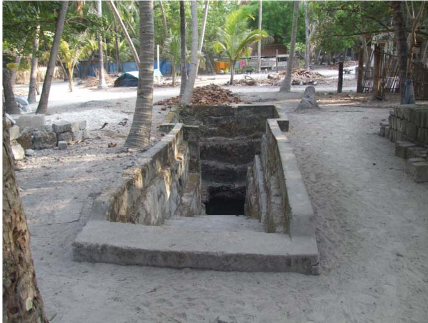
Need for renovation of such ponds under MGNREGA
