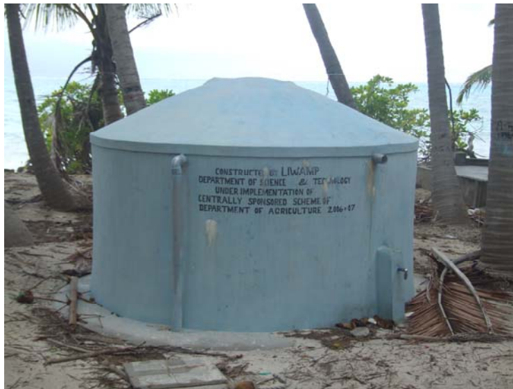
Scope for similar water conservation works under MGNREGS
