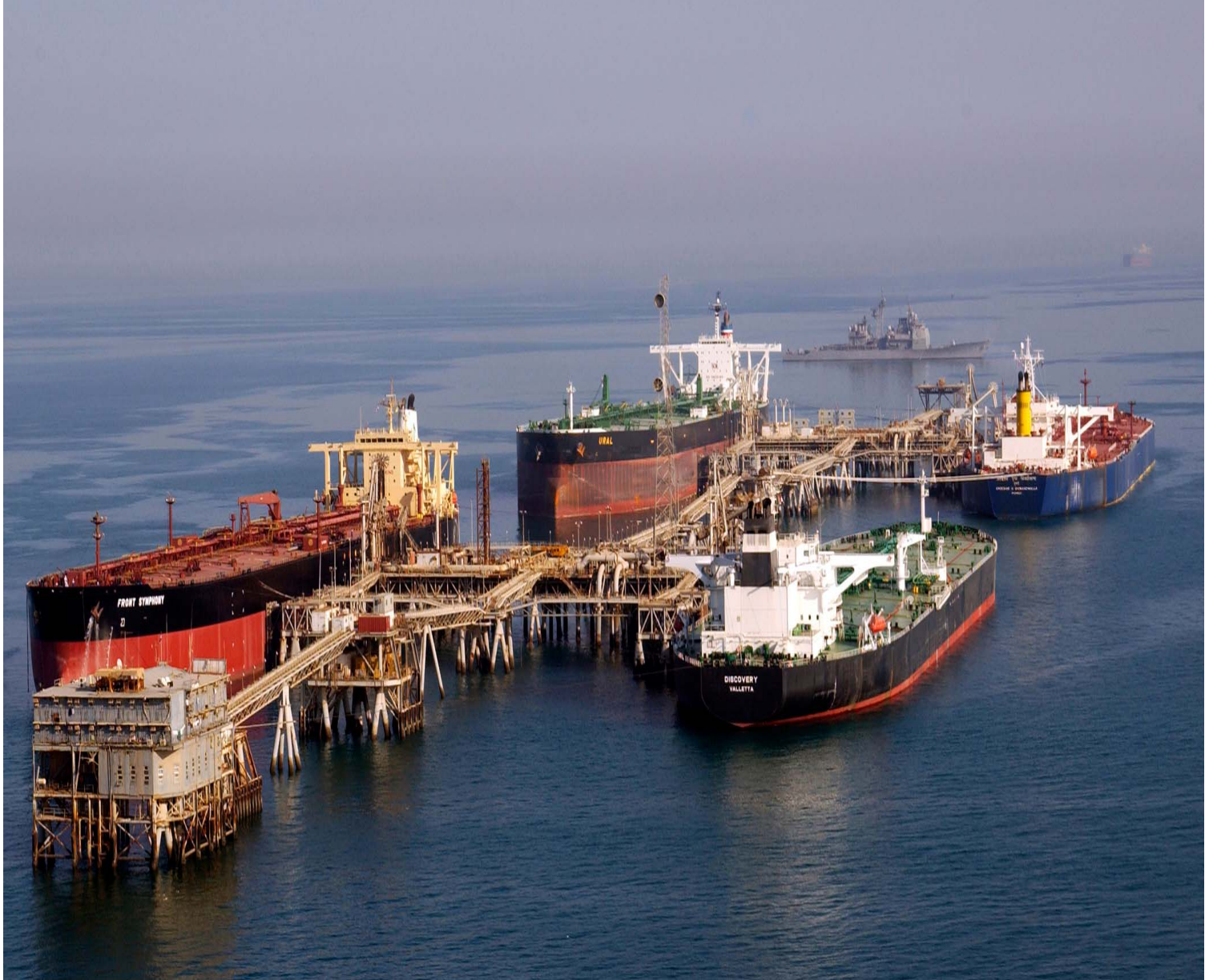
Site Photo 6. Four tankers berthed at ABOT (Photo courtesy of USACE)
