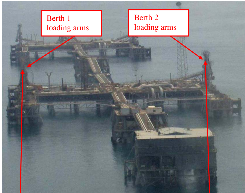
Site Photo 7. Location of Berths 1 and 2 loading arms (Photo courtesy of USACE)
