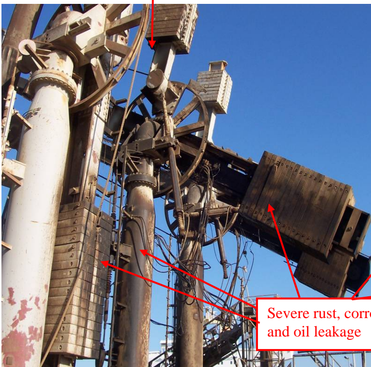
Site Photo 8. Previous condition of Berth 1 loading arm
