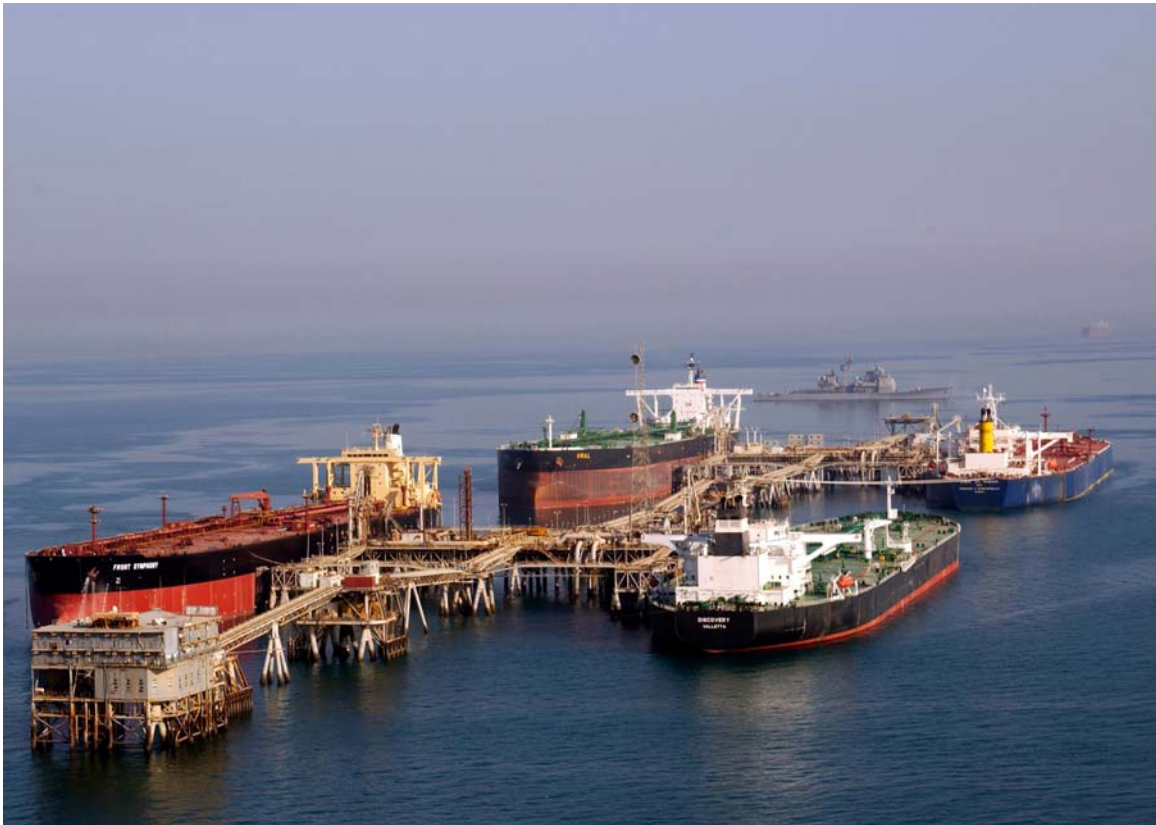
Site Photo 1. Aerial view of ABOT's four berths (Photo courtesy of USACE)
