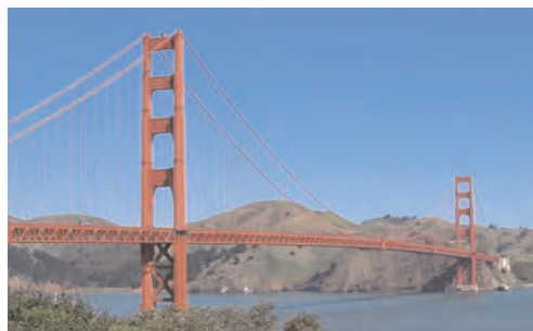
Golden Gate Bridge, San Francisco
