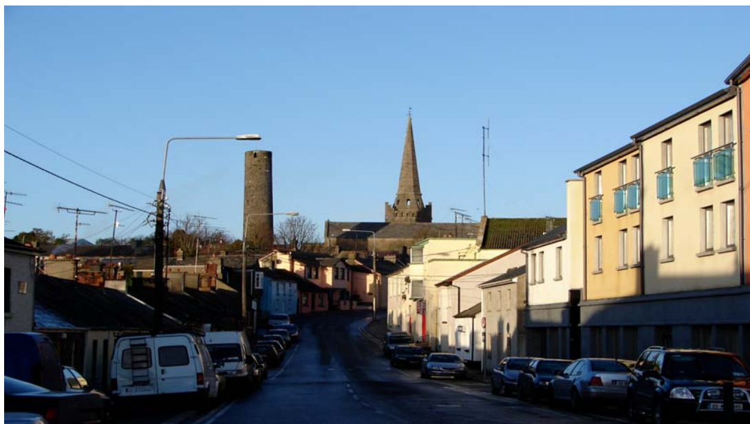
View 5.2.5 from the junction of Bective St, Farrell St and Suffolk St looking back toward the tower
