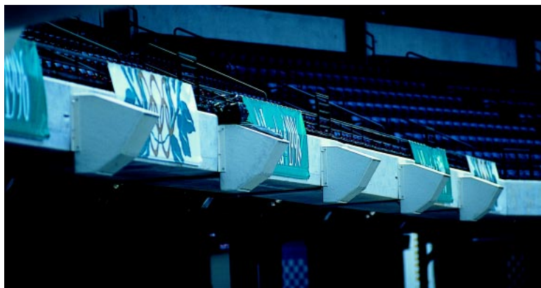
AOS90 LOUDSPEAKERS INSTALLED IN ATLANTA OLYMPIC STADIUM. THEY WERE INSTALLED IN THE PORTION OF THE STADIUM WHICH TODAY IS CALLED TURNER FIELD AND SERVES AS THE HOME TO MAJOR LEAGUE BASEBALL'S ATLANTA BRAVES.
