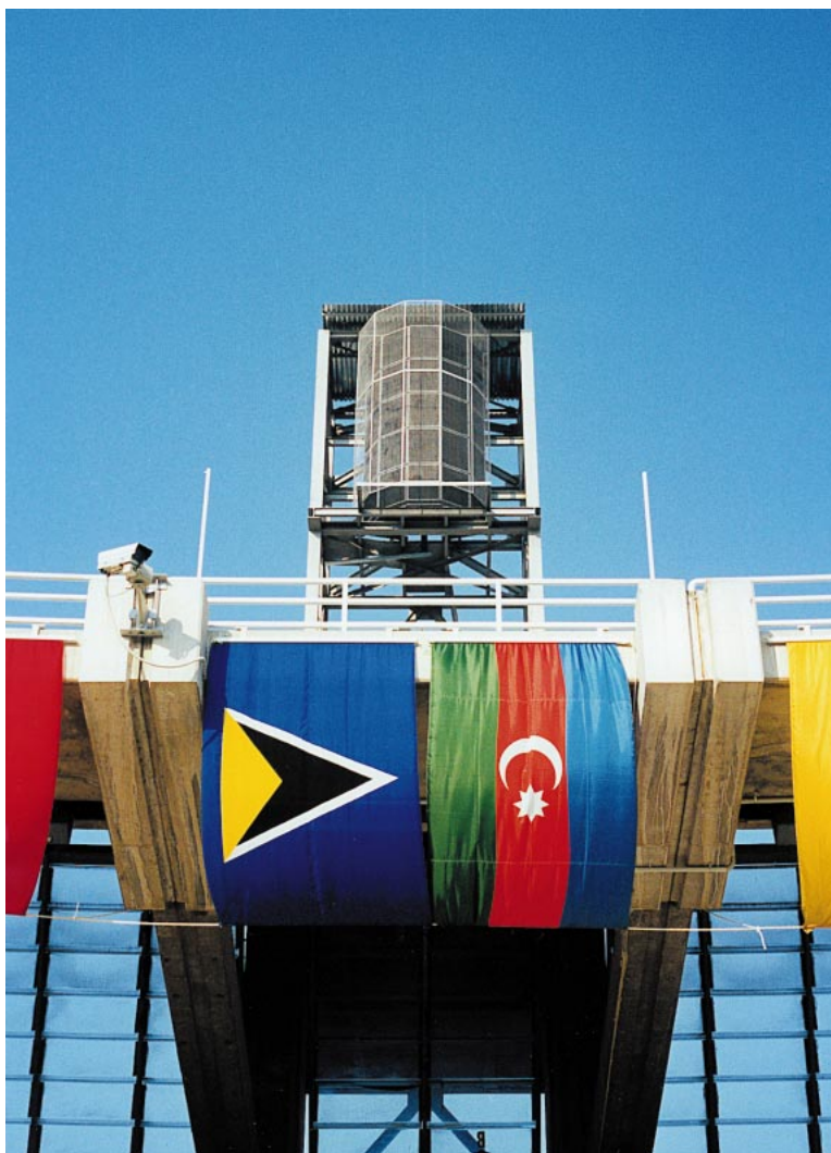
THE KF900 SERIES ARRAY INSTALLED AT OLYMPIC STADIUM, ATHENS, GREECE.
