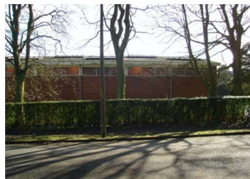
Modern Sports Centre buildings are out of character with the area though the trees mitigate the effect
