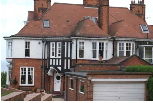
Norbury/Moor End, Weaponness Drive an eclectic mix of brick, render, 'half timbering' with highly detailed doors and eaves I
