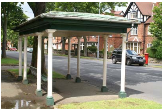
Cast iron shelter, Filey Road
