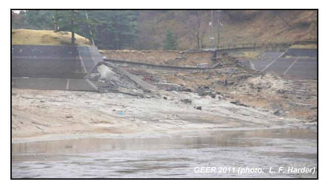
Figure 24: View of Upstream Slide in Fujinuma Auxiliary Dam from Empty Reservoir Area (N37.3011°, E140.1933°, April 23, 2011)
