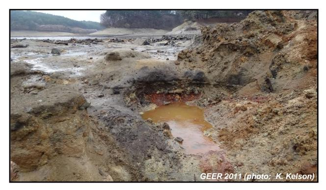
Figure 21: View of Spring within Tuff Bedrock Immediately Below Black Organic Foundation Residual Soil Exposed within Breach of Fujinuma Main Dam (N37.3017°, E140.1953°, April 23, 2011)
