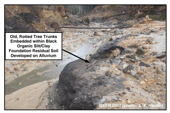
Figure 16: View of Black Organic Foundation Residual Soil Exposed in Eroded Channel Downstream of Breach in Fujinuma Main Dam (N37.3022°, E140.1959°, April 23, 2011)
