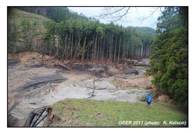
Figure 33: View of Breach Flow Path within Natural Drainage Channel Below Breach in Fujinuma Main Dam (N37.3025°, E140.1961°, April 23, 2011)
