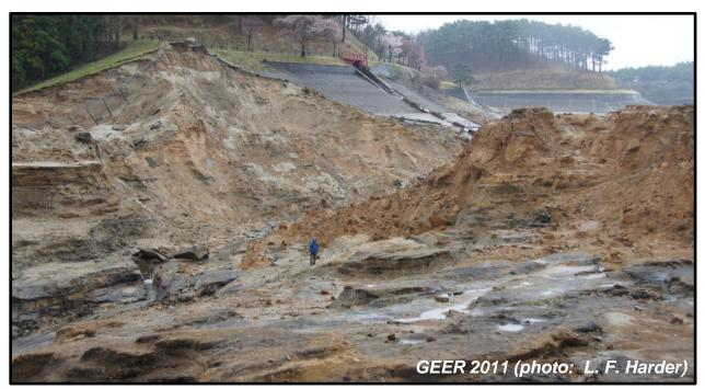
Figure 10: View of Breach in Fujinuma Main Dam from Left Abutment Looking Upstream (N37.3021°, E140.1952°, April 23, 2011)
