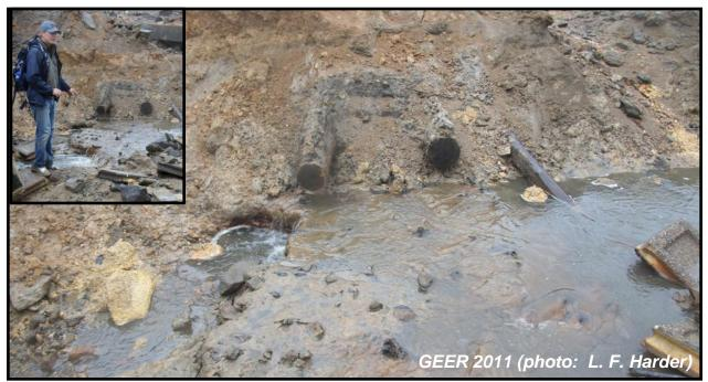
Figure 20: View of Timber Exposed in Embankment Debris Overlying Tuff Bedrock within Breach in Fujinuma Main Dam (N37.3019°, E140.1954°, April 23, 2011)
