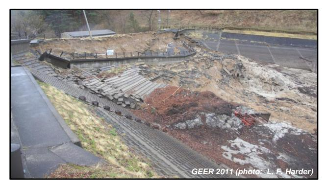
Figure 25: View of Upstream Slide in Fujinuma Auxiliary Dam from Location Upstream of Auxiliary Dam Left Abutment (N37.3011°, E140.1933°, April 23, 2011)
