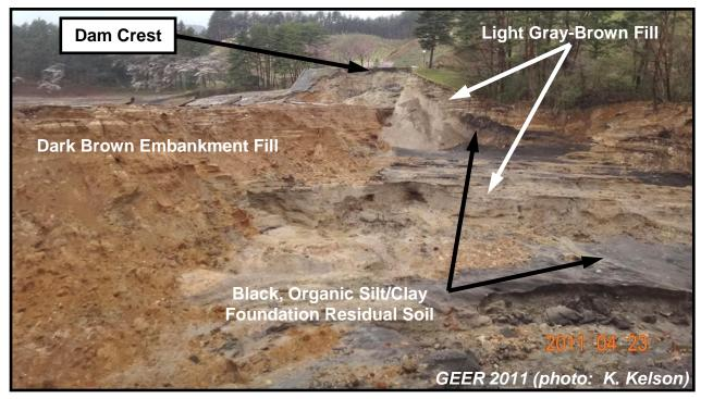
Figure 12: View of Eroded Downstream Slope of Fujinuma Main Dam from Right Abutment – Note Uniform Top Surface of Dark Brown Embankment Fill Zone Below Dam Crest (N37.3020°, E140.1959°, April 23, 2011)
