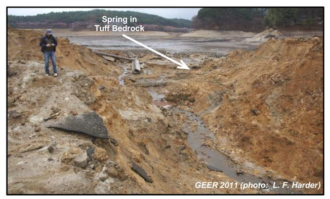
Figure 9: View of Breach in Fujinuma Main Dam Looking Upstream towards Empty Reservoir (N37.3021°, E140.1958°, April 23, 2011)
