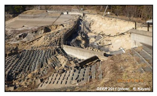
Figure 28: View of Upstream Slide in Fujinuma Auxiliary Dam from Auxiliary Dam Right Abutment (N37.2990°, E140.1952°, April 5, 2011)
