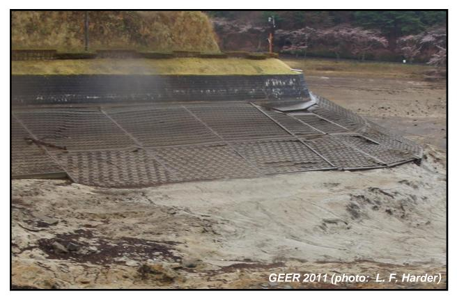
Figure 31: View of Slope Distress in Revetted Reservoir Rim Slope Upstream of Fujinuma Auxiliary Dam Right Abutment (N37.2990°, E140.1945°, April 23, 2011)
