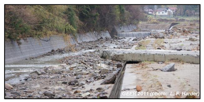
Figure 36: Views of Erosion and Damage within River Channel in Naganuma Below Breach in Fujinuma Main Dam (N37.3062°, E140.2064°, April 23, 2011)
