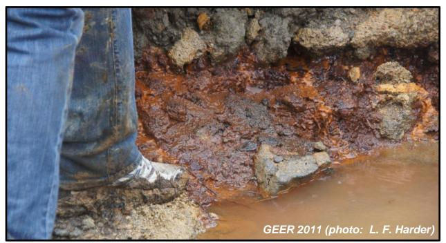
Figure 22: View of Spring within Tuff Bedrock Immediately Below Black Organic Foundation Residual Soil Exposed within Breach in Fujinuma Main Dam (N37.3017°, E140.1953°, April 23, 2011)
