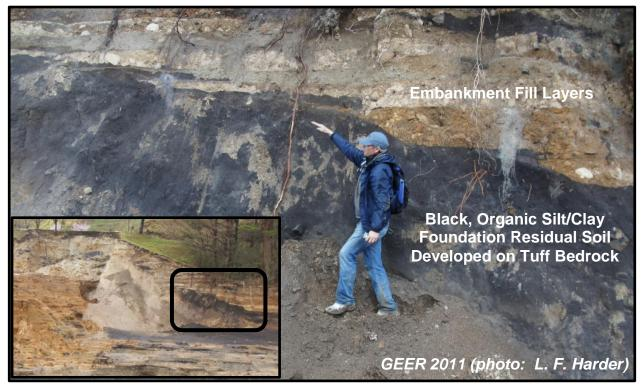
Figure 14: View of Fujinuma Dam Embankment Fill Layers On Top of Black Organic Foundation Residual Soil Exposed within Downstream Slope at Left Abutment (N37.3024°, E140.1951°, April 23, 2011)
