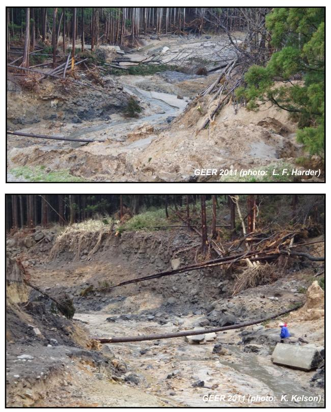
Figure 34: Views of Downstream Erosion within Natural Drainage Channel Below Breach in Fujinuma Main Dam (N37.3025°, E140.1961°, April 23, 2011)
