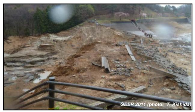
Figure 11: View of Breach in Fujinuma Main Dam from Left Abutment (N37.3024°, E140.1946°, April 23, 2011)
