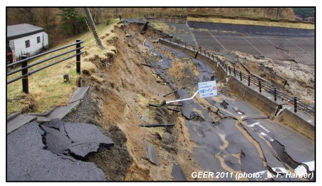
Figure 26: View of Upstream Slide in Fujinuma Auxiliary Dam from Left Abutment (N37.2995°, E140.1956°, April 23, 2011)
