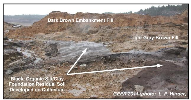
Figure 13: View of Eroded Downstream Slope of Fujinuma Main Dam from Downstream Toe – Note Uniform Top Surface of Dark Brown Embankment Fill Zone below Dam Crest and Lighter Gray-Brown Embankment Fill Overlying Black Organic Foundation Residual Soil (N37.3023°, E140.1955°, April 23, 2011)
