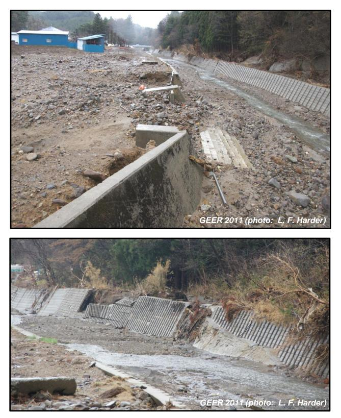
Figure 37: Views Looking Downstream of Debris, Erosion, and Damage within River Channel in Naganuma below Breach in Fujinuma Main Dam (N37.3044°, E140.2076°, April 23, 2011)
