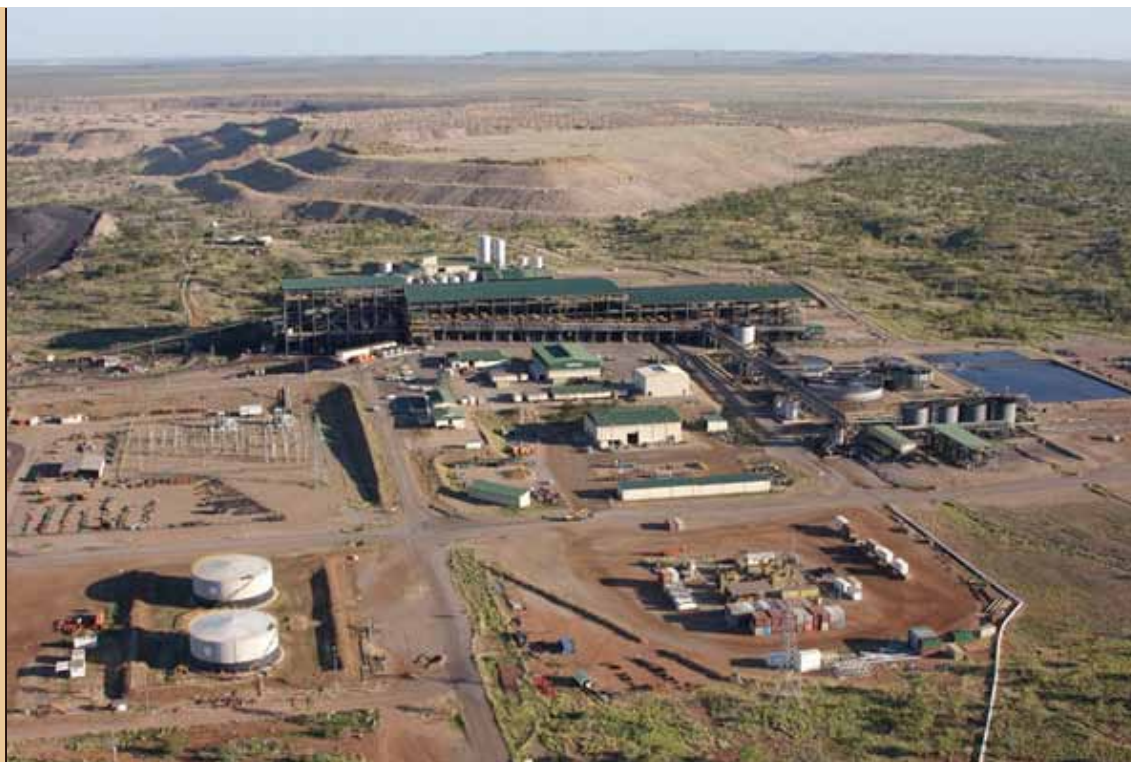
Surface facilities Century zinc-lead mine, north Queensland (Minerals and Metals Group Ltd)
