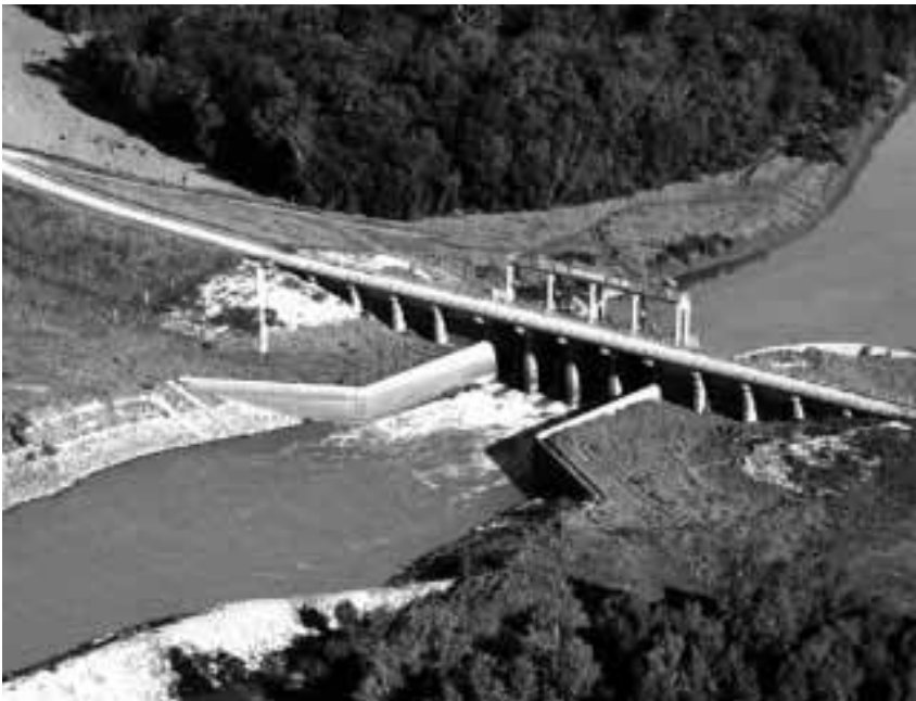
A HYDRAULIC PUMPING PLANT, PICTURED BELOW, CAN DRAIN THOUSANDS OF ACRES OF WETLANDS IN A SHORT TIME. THE PROPOSED YAZOO PUMP WOULD BE THE WORLD’S LARGEST.
