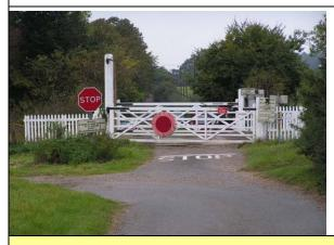
**User-worked crossing with miniature warning lights** (**UWC-MWL**) This crossing has gates or full lifting barriers, which the user must operate prior to crossing. Red/green miniature warning lights, operated by the approach of trains, inform the user whether it is safe to cross.
