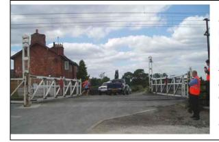
**Manually controlled gate (MCG)** This crossing is equipped with gates, which are manually operated by a signaller or crossing keeper either before the protecting signal can be cleared, or with the permission of the signaller or signalling system. At the majority of these crossings, the normal position of the gates is open to road traffic, but on some quiet roads the gates are maintained 'closed to the road' and opened when required if no train is approaching.
