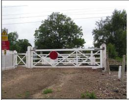
**User-worked crossing with telephone (UWC-T)** These are similar to the standard user worked crossing, but a telephone is provided. In some circumstances (for example when crossing with livestock or vehicles) the user must contact the signaller for permission to cross, and report back when they are clear of the track. They are provided where visibility of approaching trains is limited, or the user needs to move livestock over the railway on a regular basis.
