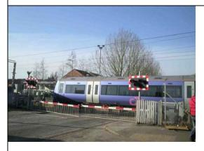
Manually controlled barrier protected by closed circuit television (MCB-CCTV) Similar to MCB crossings, except that a closed circuit television (CCTV) is used to monitor and control the crossing from a remote location.
