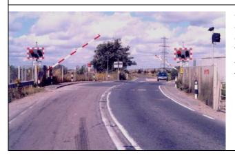
Automatic barrier locally monitored (ABCL) As far as the road user is concerned, this crossing looks identical to an AHB crossing. The difference is that train drivers must ensure that the crossing is clear before passing over it. Train speed is limited to 55mph or less.
