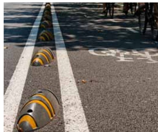
Traffic separators for cycle lanes made from post-consumer PVC waste
